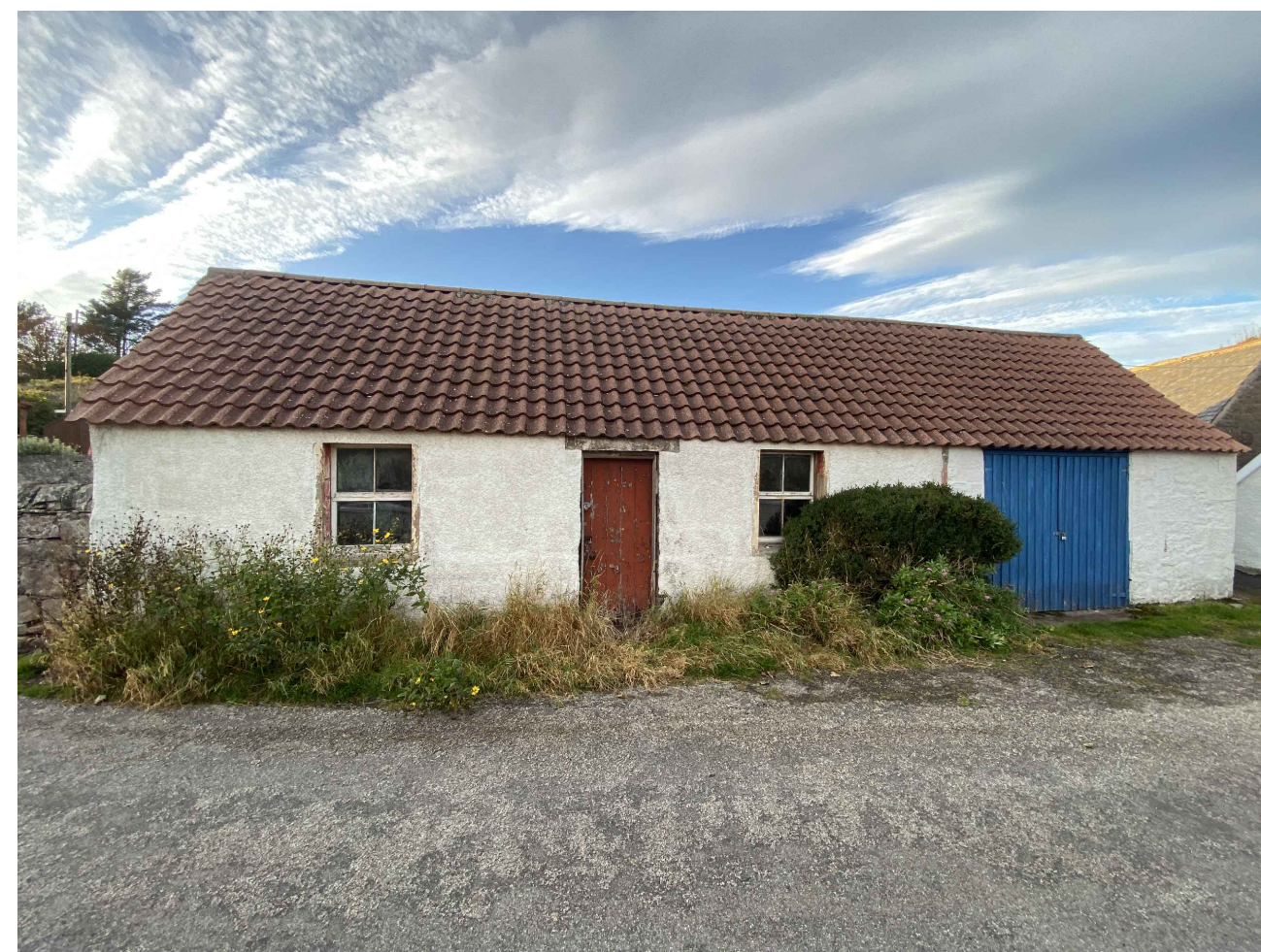
PHOTO OF EXISTING
