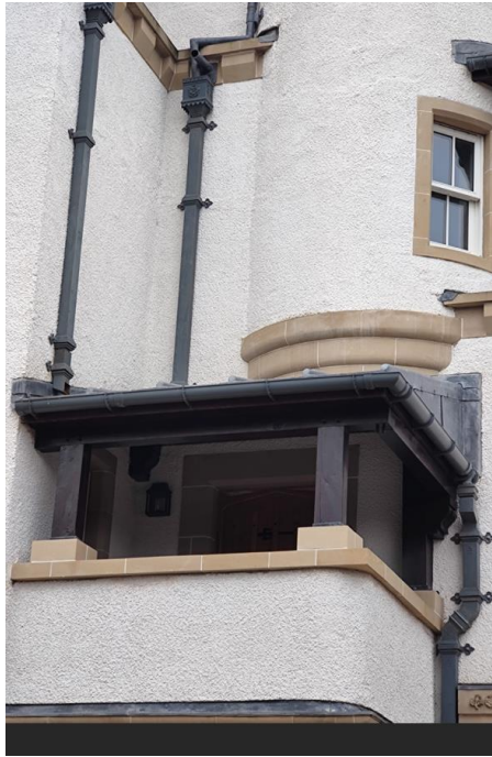
Figure 5 – traditional stone, render and leadwork – extension SE elevation first and second floors – the modulation of planes
