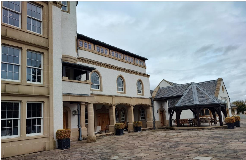
Figure 22– southeastern elevation from terrace looking towards north east.
