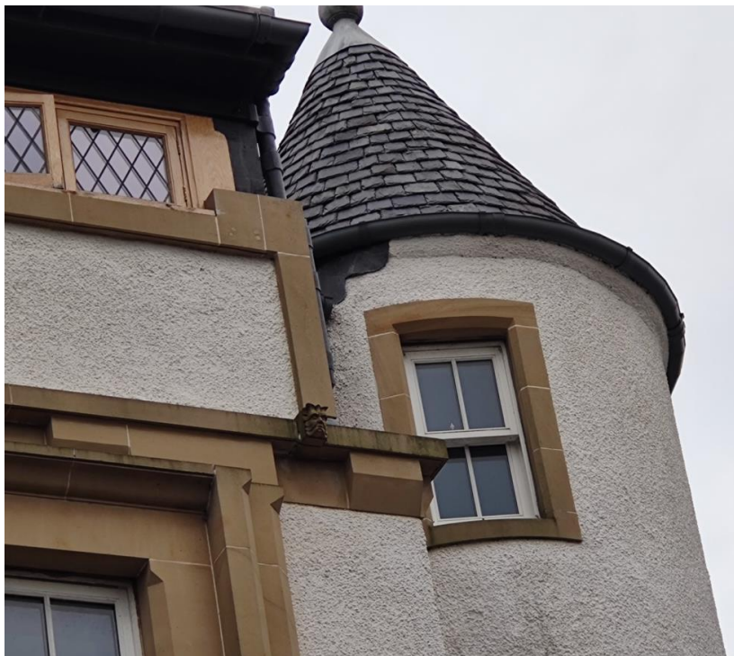
Figure 20 – south eastern elevation – enclosed terrace at third floor
