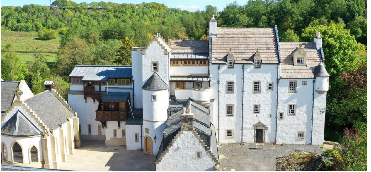
Figure 13 – Aiket Castle part elevation to northwest ; enclosed roof terraces; multipurpose 2 nd floor room to left, third floor link corridor abutting tower house gable.
