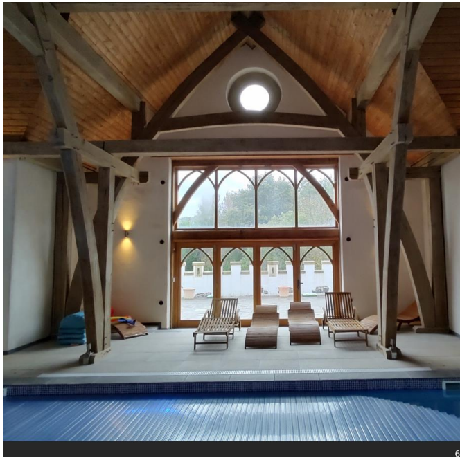
Figure 9-10 Pool building with exposed oak frame
