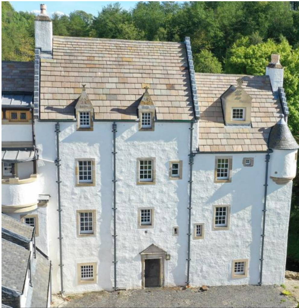
Figure 14 – Aiket Castle northeastern elevation-existing/ new junction
