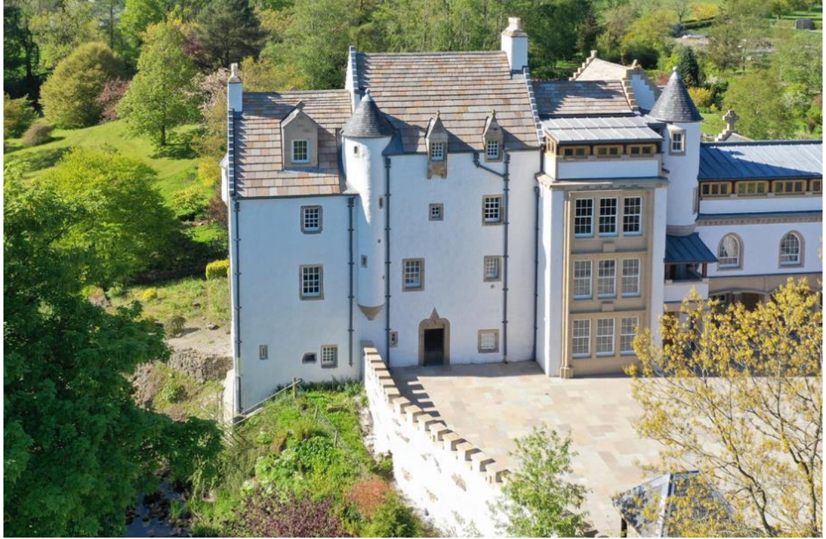
Figure 15 – Aiket Castle southeastern part elevation – existing/ new junction , enclosed terraces at second and third floor
