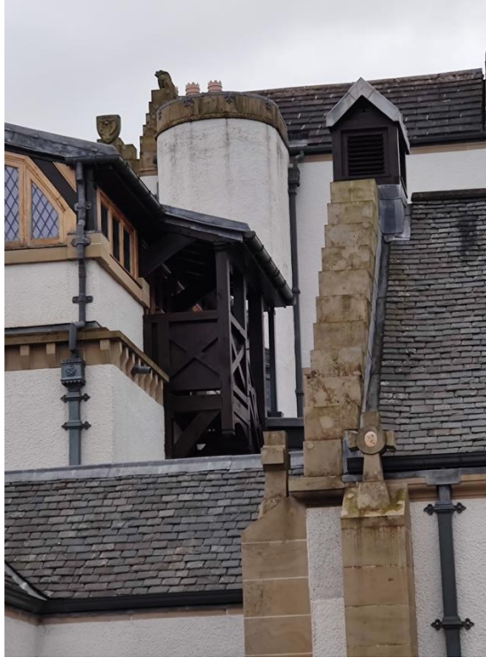
Figure 19 – looking to north east elevation from pool/ chapel courtyard -stepping down in scale, layering of planes and materials
