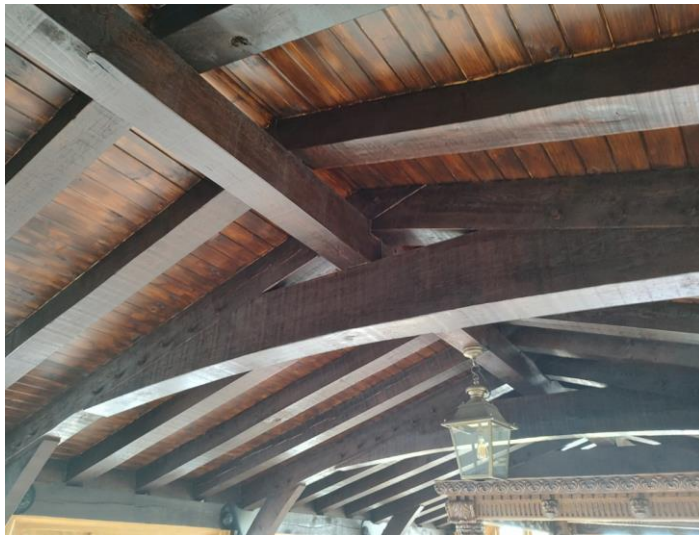
Figure 26– internal timber detailing – enclosed terraces
