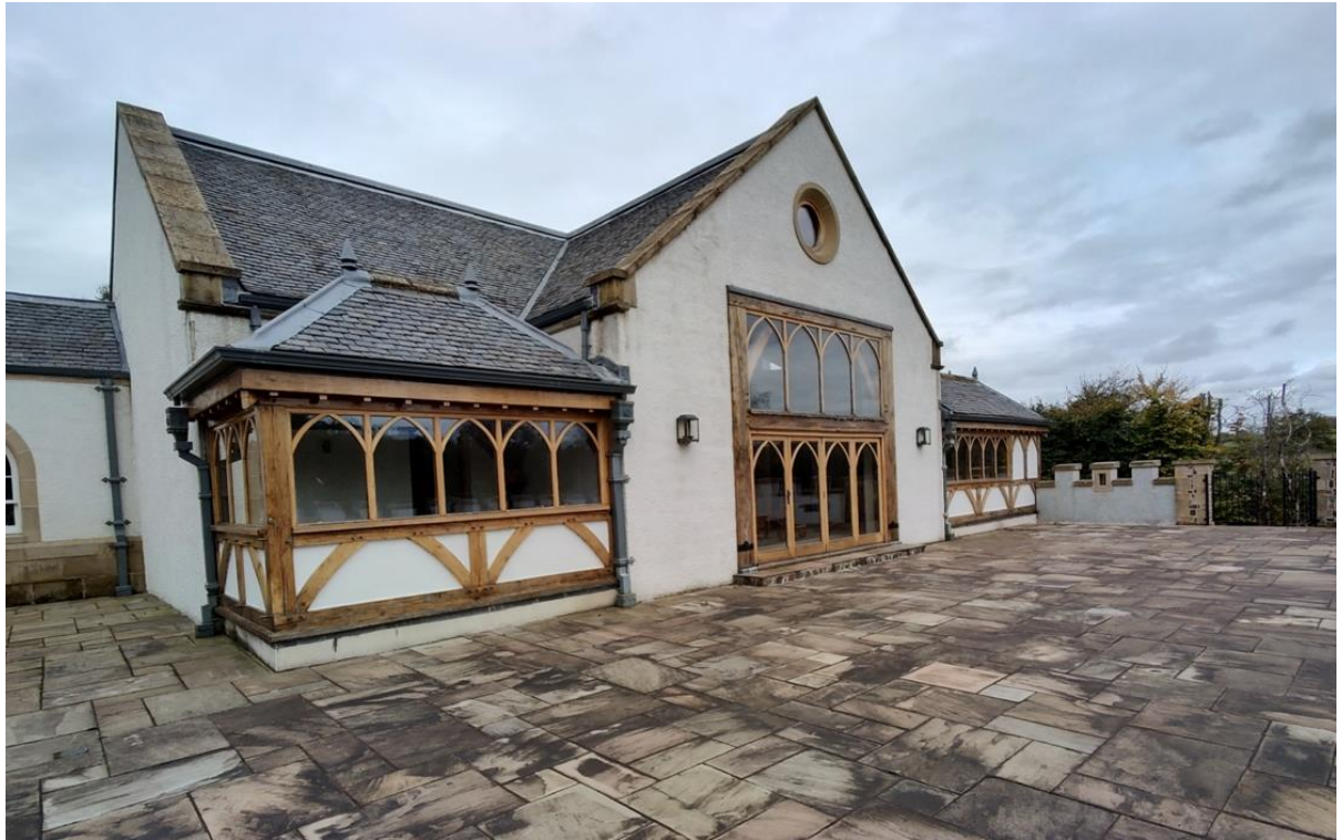
Figure 16 – Southeastern elevation of pool building. New bays reduce scale and refer to other timber structure
