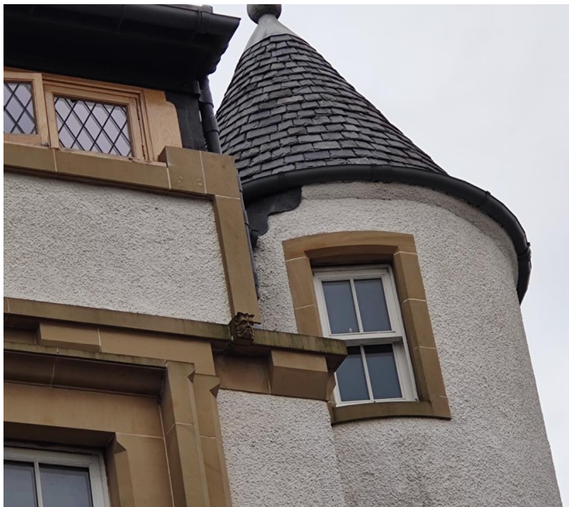
Figure 31 – south eastern elevation – enclosed terrace at third floor
