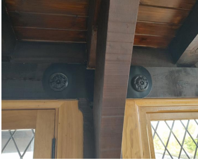
Figure 36- internal timber detailing – enclosed terraces
