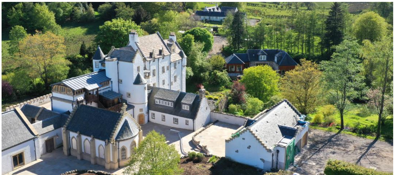
Figure 23 – Aiket Castle northeastern elevation-garage bays, pool rear fenestration, enclosed roof terrace
