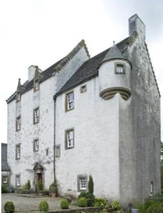
Figure 12 – north west / west gable
