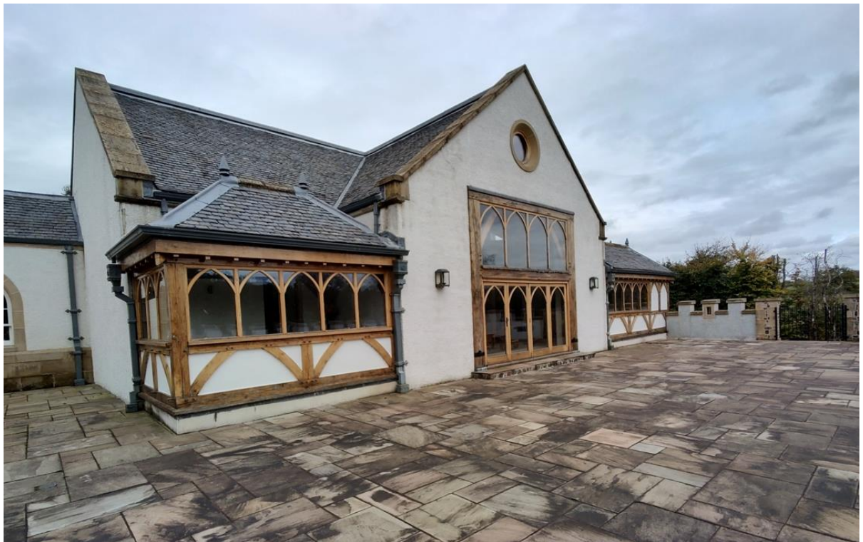
Figure 27 – Southeastern elevation of pool building. New bays reduce scale and refer to other timber structure
