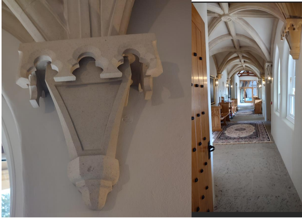
Figures 15-16 - internal stone corbel and vaulted cloister link.
