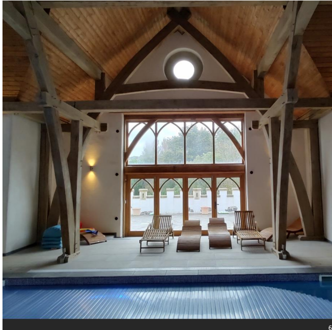
Figure 20-21 Pool building with exposed oak frame
