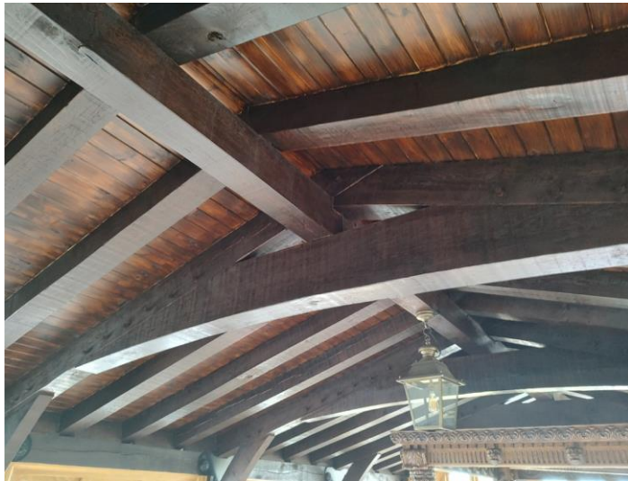
Figure 37- internal timber detailing – enclosed terraces
