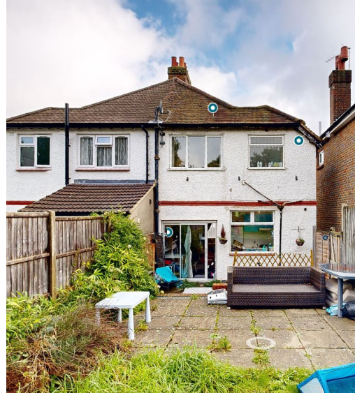
Existing Rear facade
