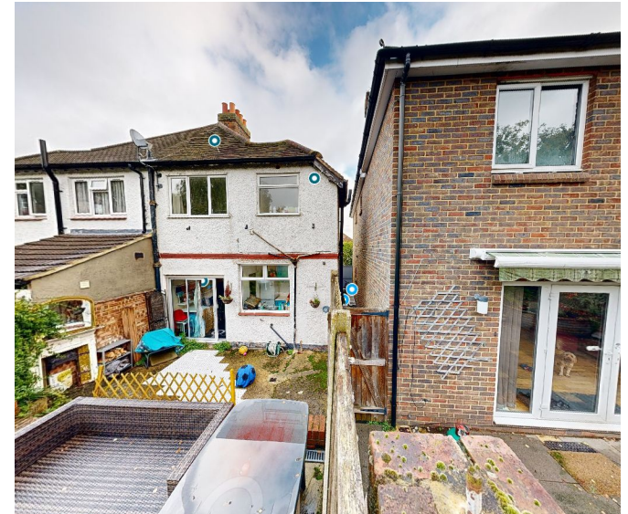
Existing Rear facade and neighbouring context
