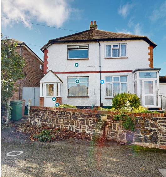
Existing Front facade
