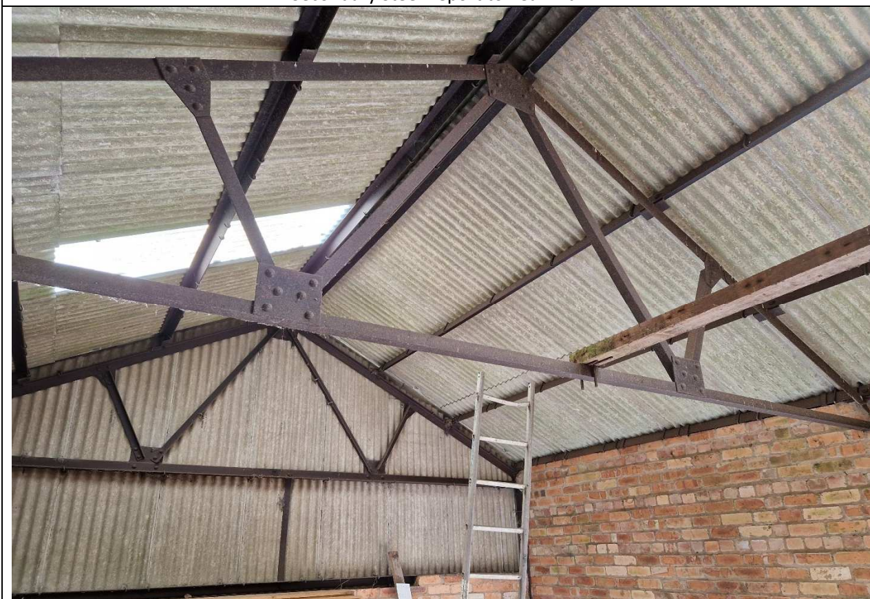
Typical Trusses Supporting Existing Roof
