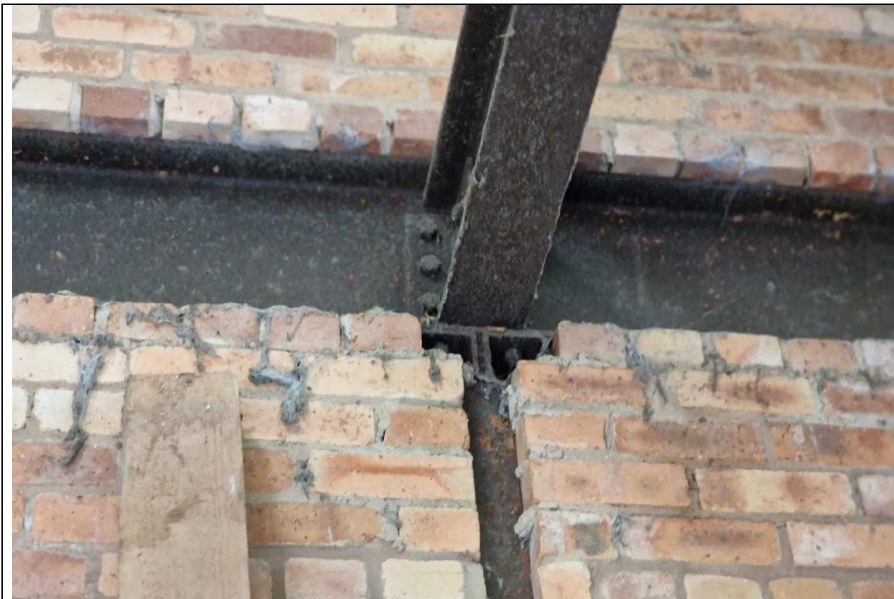
Secondary Steel Report to Rear Wall
