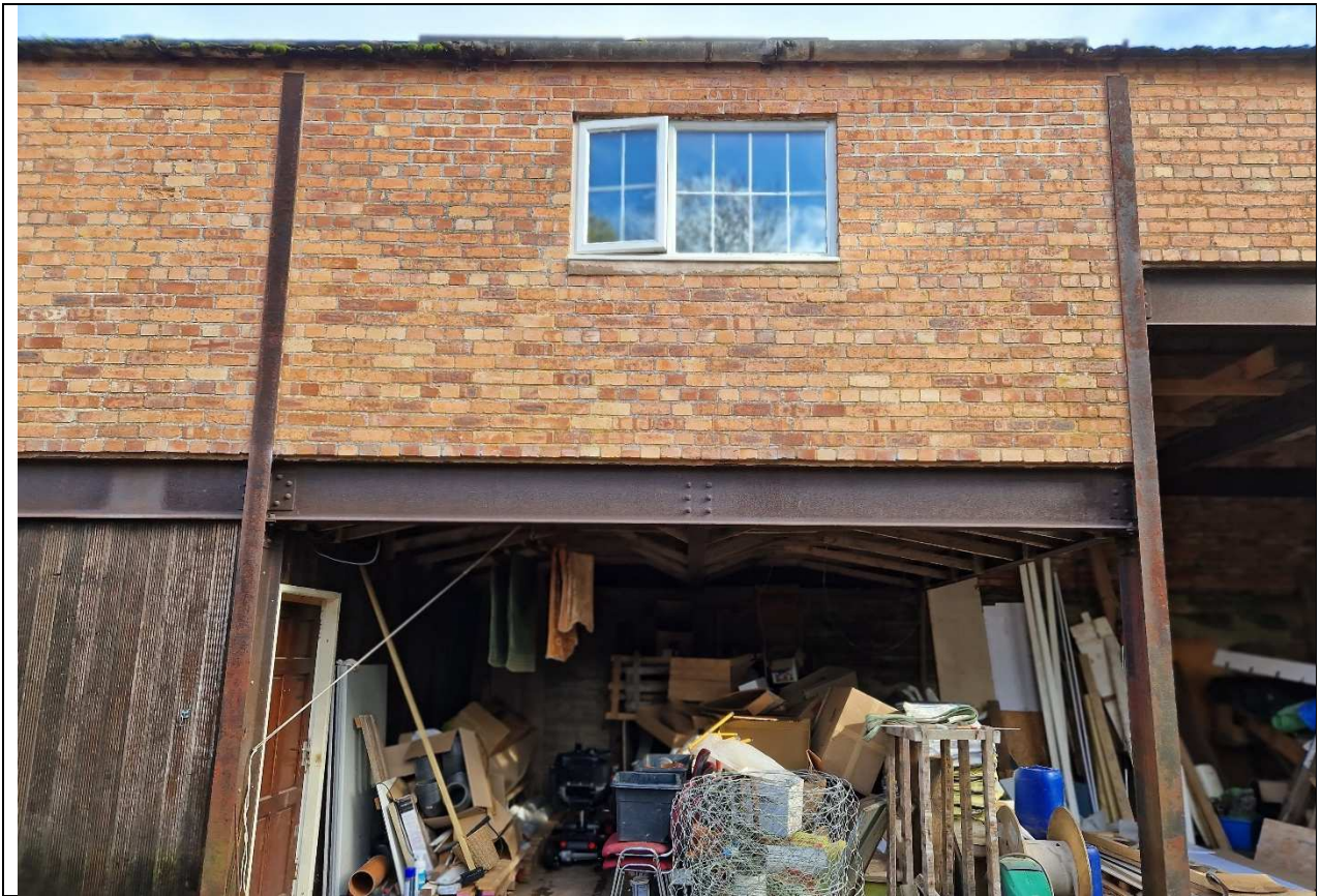
Typical Steel Frame to Front of Building
