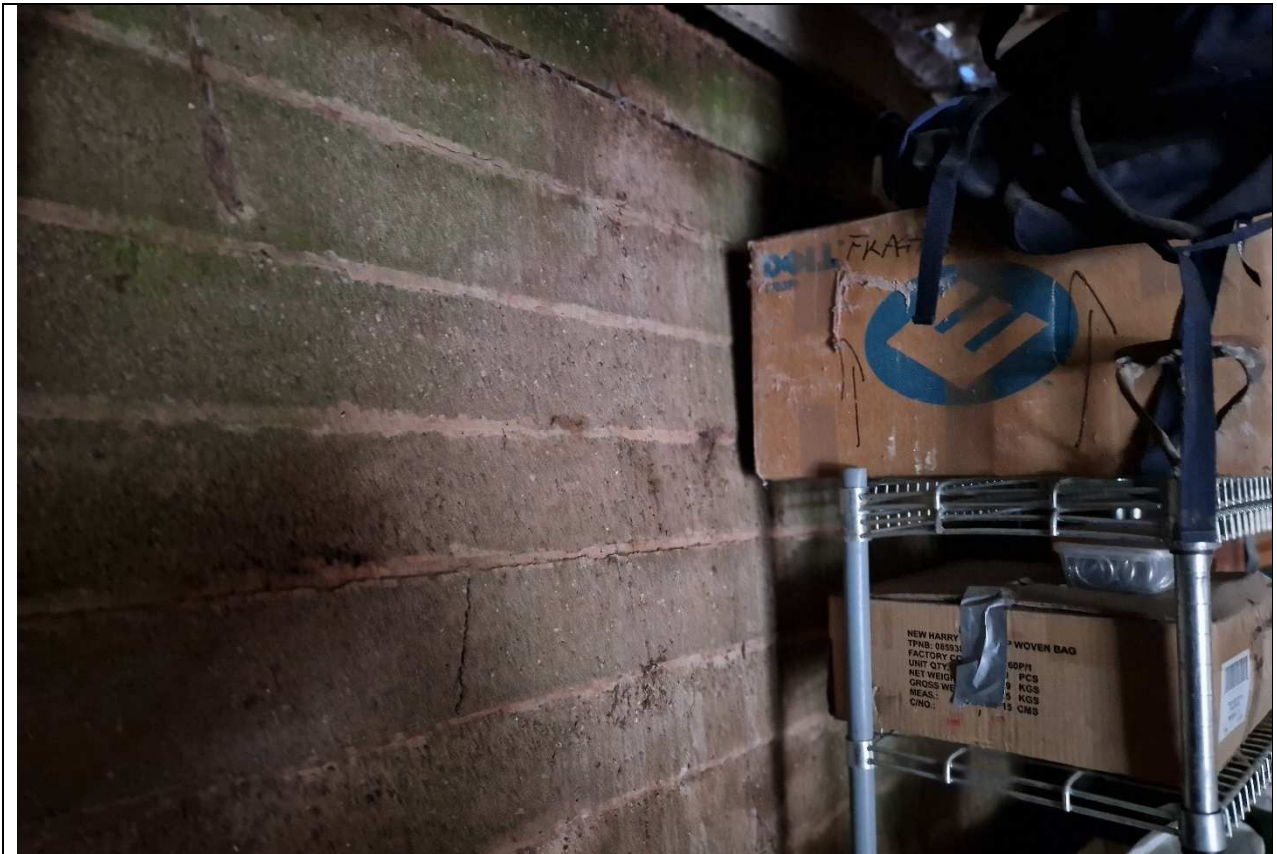
Retaining Wall to Left Side Wall at Ground Floor Level
