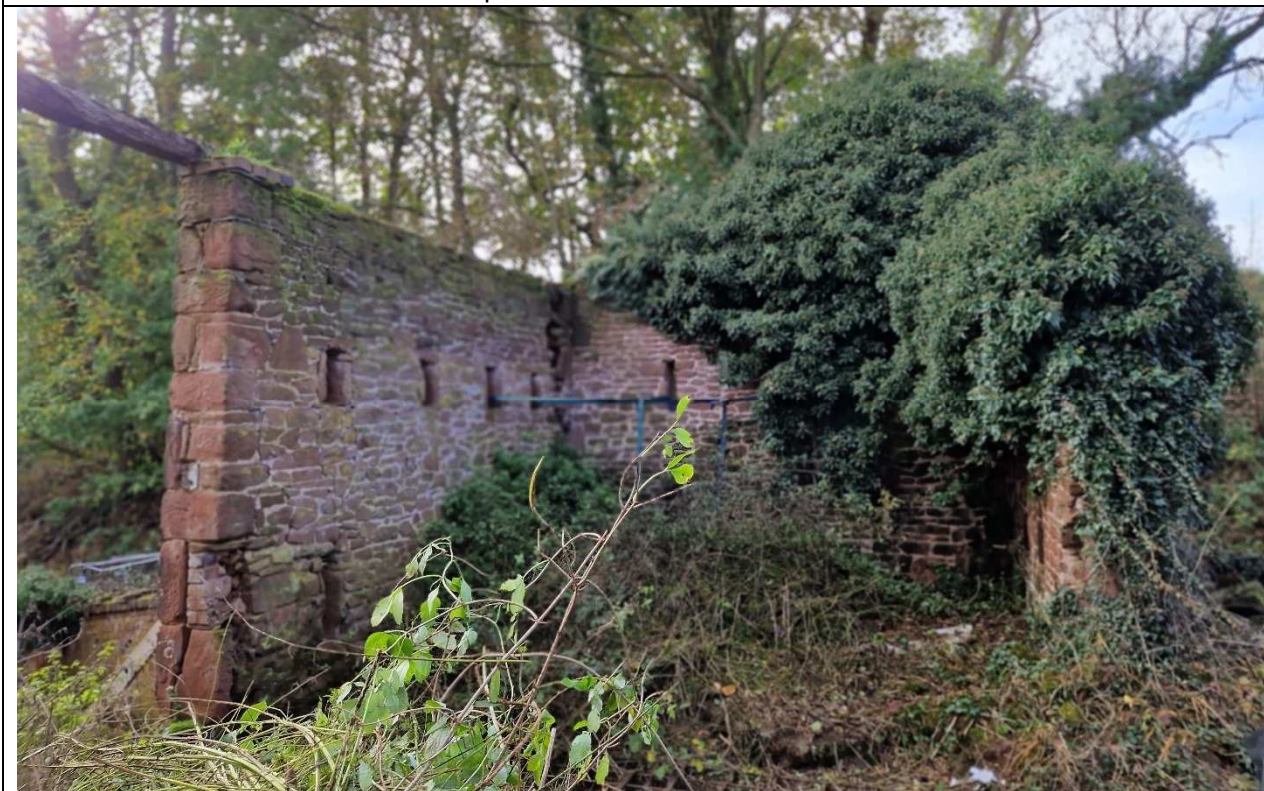
Old Barn Walls to West
