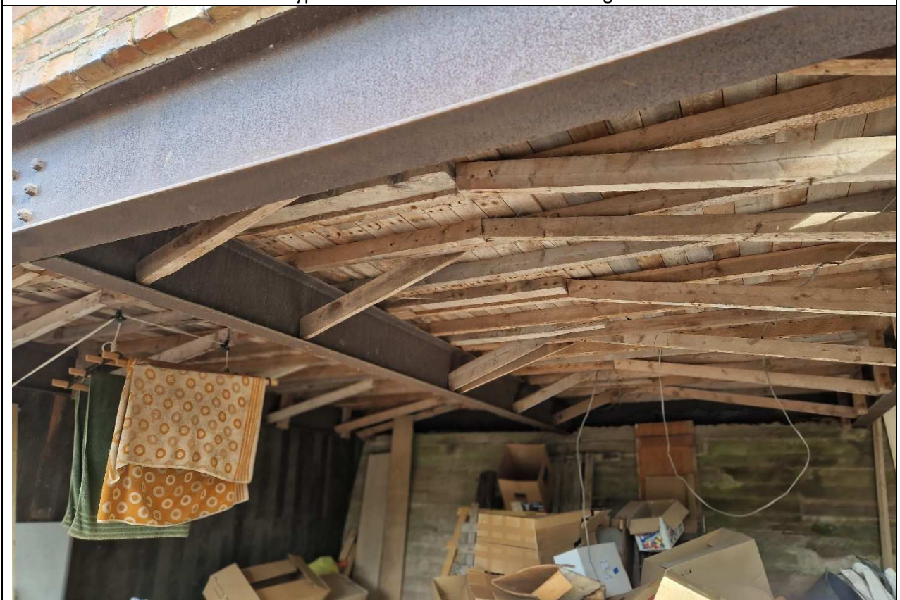
Steel Frame Support to 1 st Floor Joists
