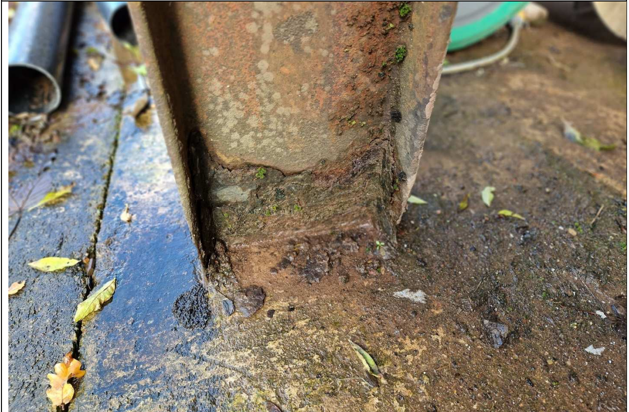
Steel Breakdown to Webs of Columns at Front
