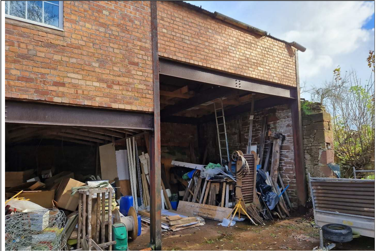
Split Level Frame at Front Right
