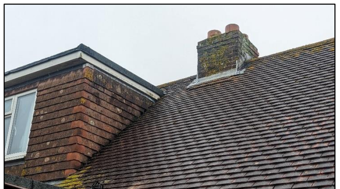
Photo 8: East facing roof. Slipped tile under chimney
