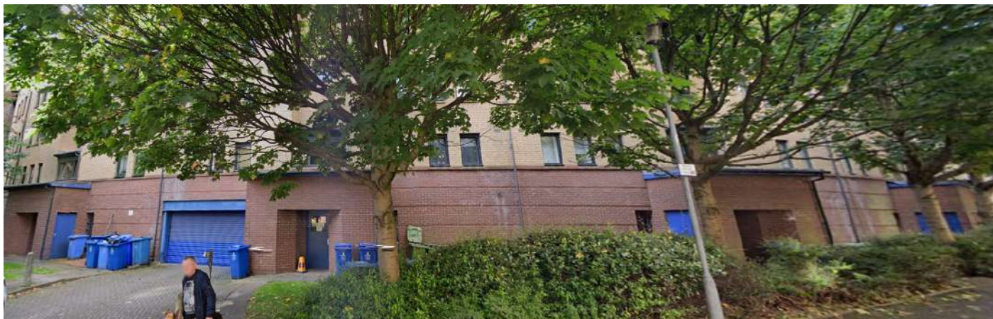
Rear Elevation of Turnbull Street
