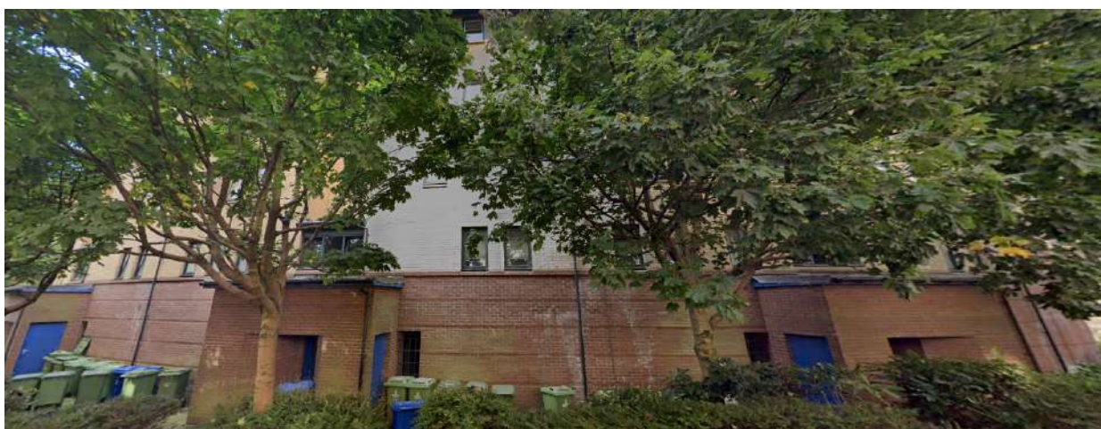
View facing South West to the Rear Elevation Centre of Curving Elevation with windows Facing North East
