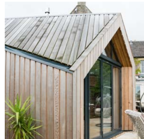
Cedar clad extension to Listed property - The Old Rectory, Buckland Dinham Abi McGillivray Architecture
