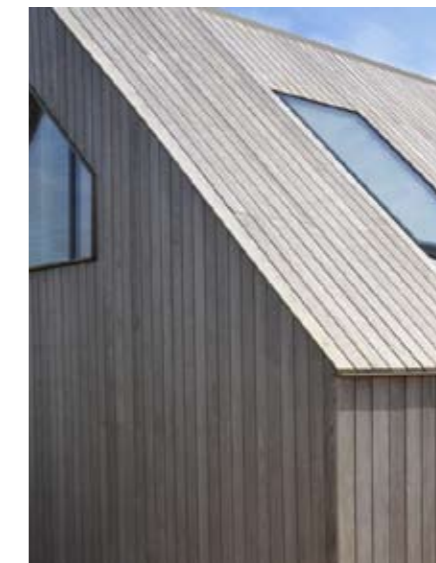
Heat treated - modified Abodo timber suitable for use as roof and wall cladding - with improve longevity and thermal performance
