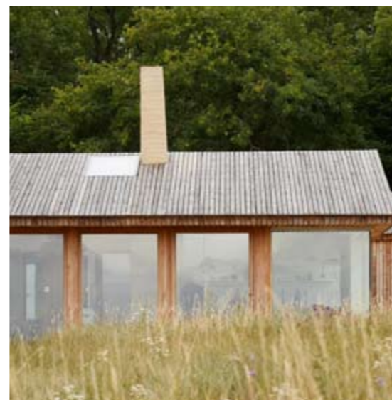
Example of timber roof cladding and eaves, (with hidden gutters) Dwelling By Hutch Design
