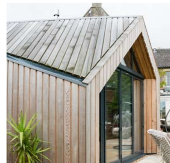
Cedar clad extension to Listed property - The Old Rectory, Buckland Dinham Abi McGillivray Architecture
