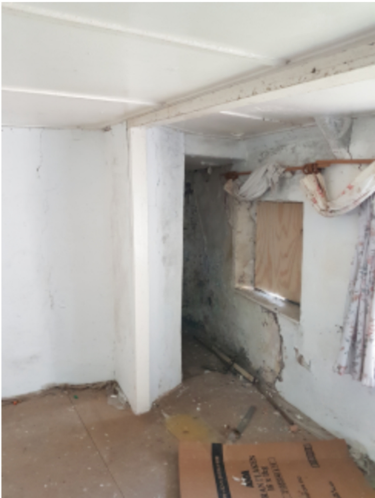
First Floor June 2018
