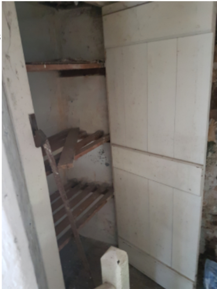
First Floor Interior June 2018
