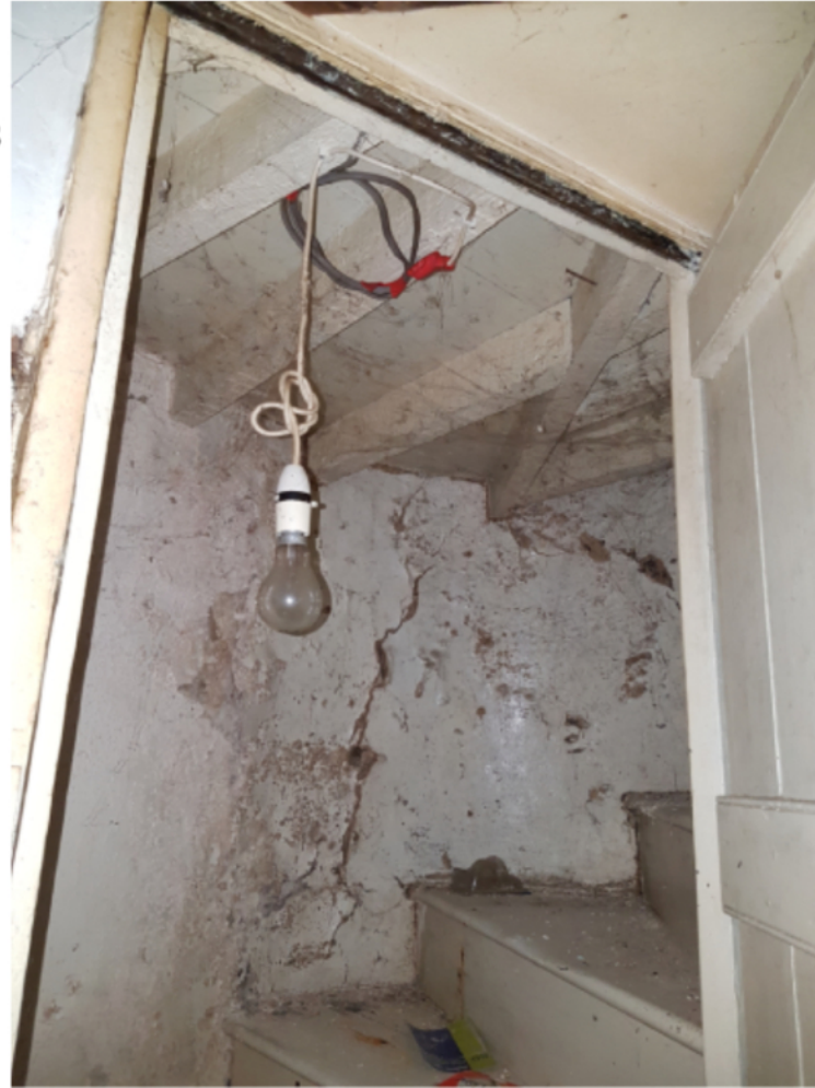
Ground Floor Interior June 2018
