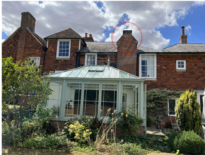
Fig 1: Rear Elevation of Laddingford House showing the existing chimney to be reinstated.
