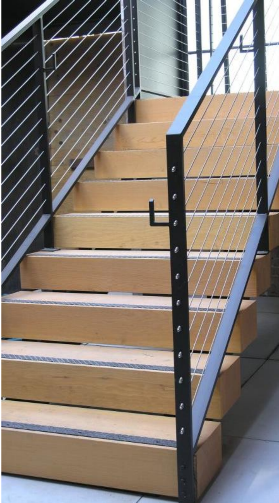
Figure 7 (Left) - Timber tread staircase, metal plate stinger, with square balustrade posts, mesh infill and timber handrail. Image © Mountain Laurel Handrails
