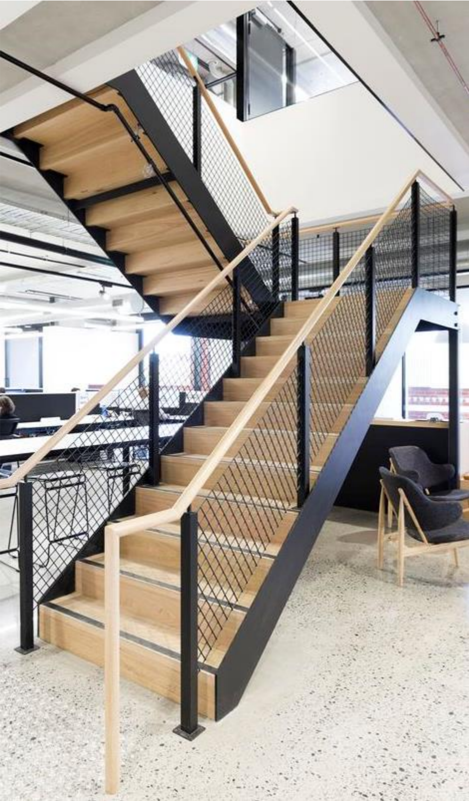
Figure 7 (Left) - Timber tread staircase, metal plate stinger, with square balustrade posts, mesh infill and timber handrail. Image © Mountain Laurel Handrails
