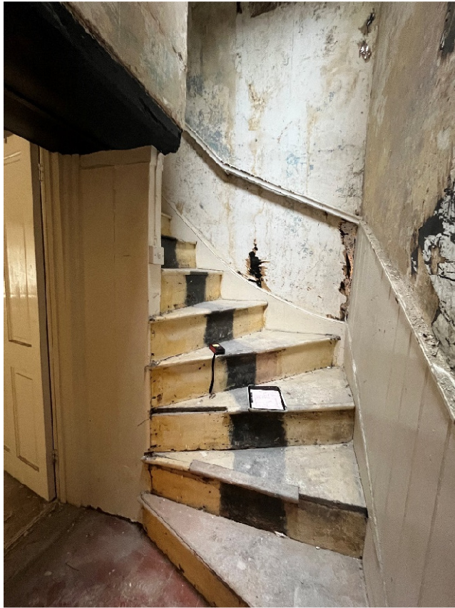
Stairs to first floor
