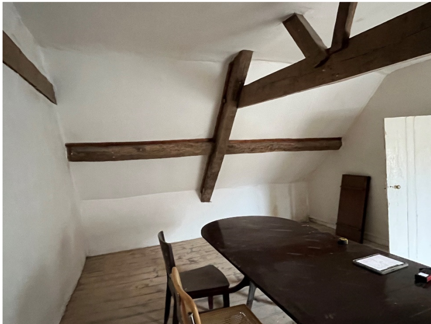
Attic rooms showing location of proposed rooflights
