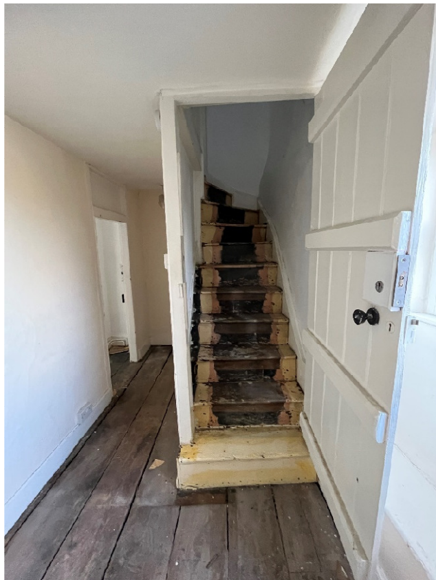
Stairs to second floor
