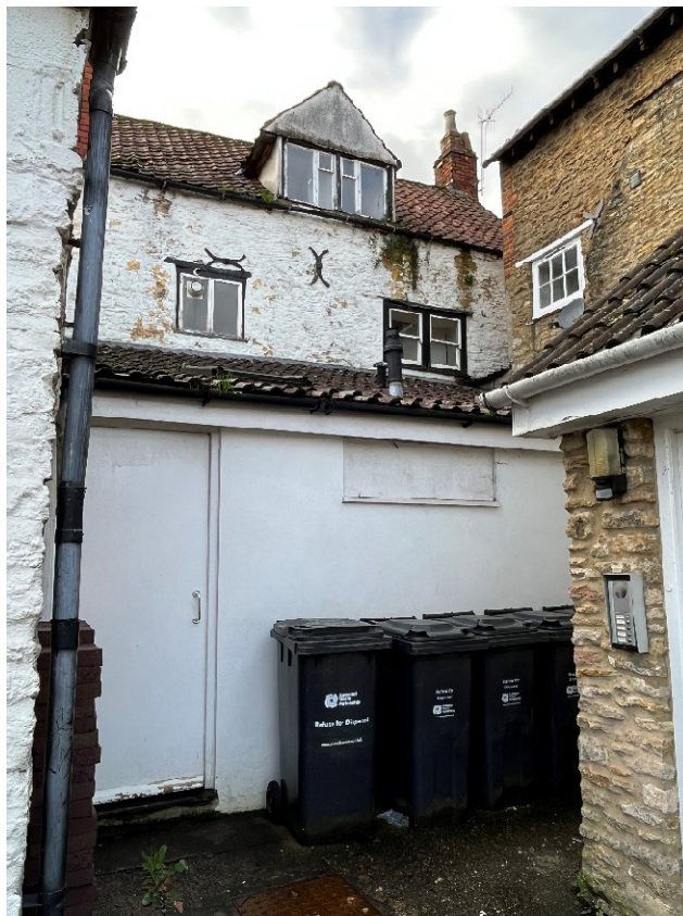
Rear of the building facing the courtyard
