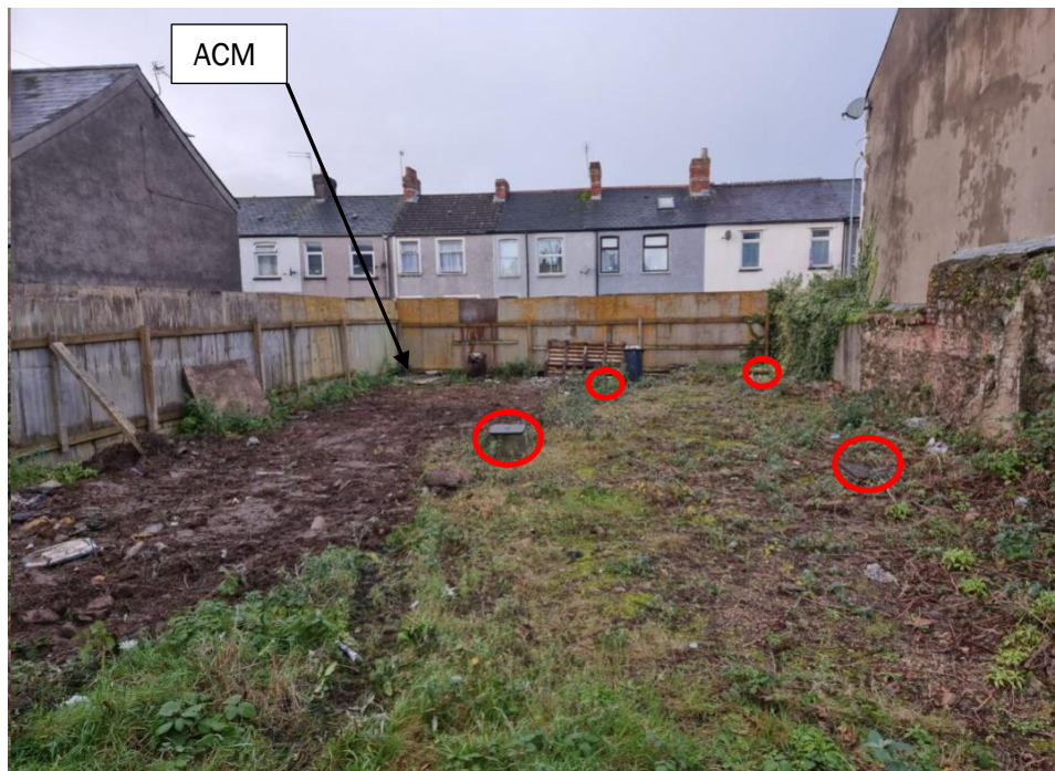
Insert 3: View of current site conditions (ESP 2023)
