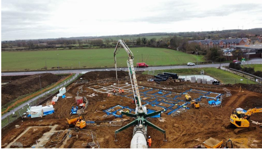
An aerial view of work progressing on the new development
