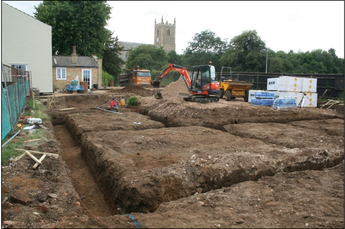
Plate 9: Overall view of house foundation trenches, looking south-west.
