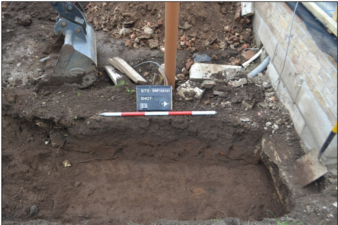
Plate 12: East facing representative section of service trench. Fig. 6, sec. 8. Scale 1 x 1m.
