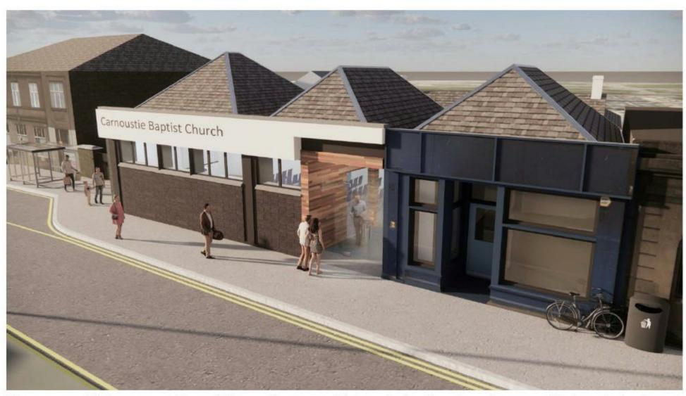
The proposal is to remove the existing entrance and 'shopwindow' and create a new timber clad entrance feature that will act as canopy and separation of the entrance and frontage elements of the building. The timber clad will cotnue into the building, helping to draw people inside and the modern appearance indicating freshness and change. New glass entrance doors and sidepanel will create a much larger and more open entrance, allowing both views and light into the building.
