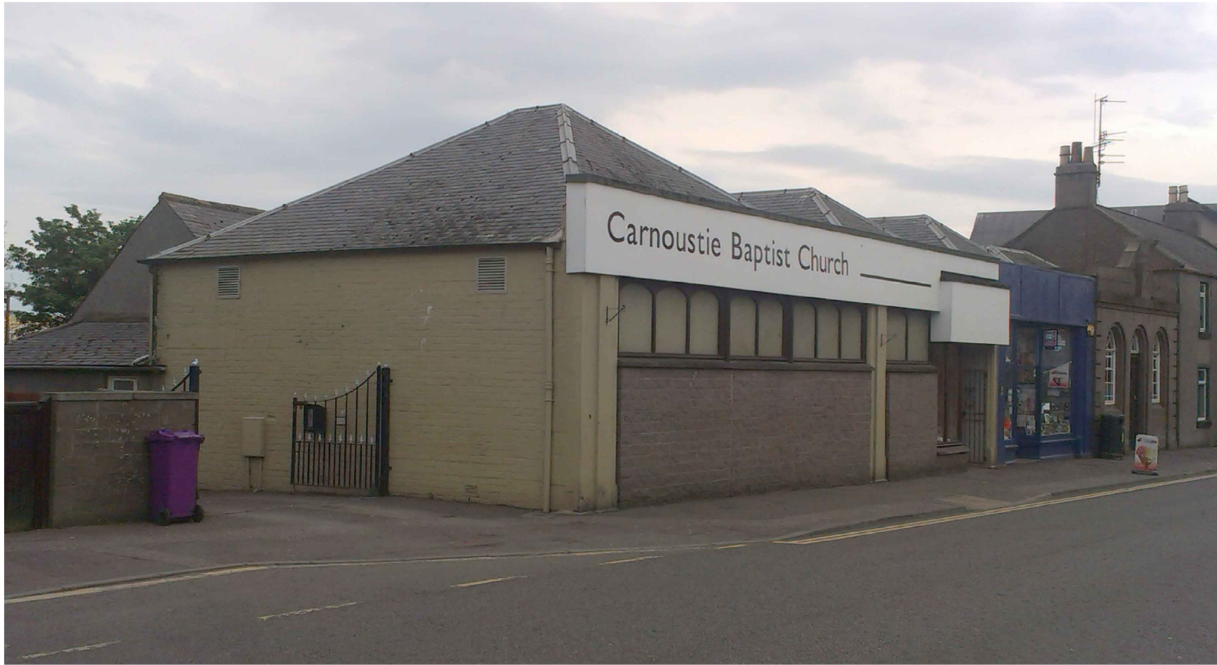
3D View 3: Frontage Existing
