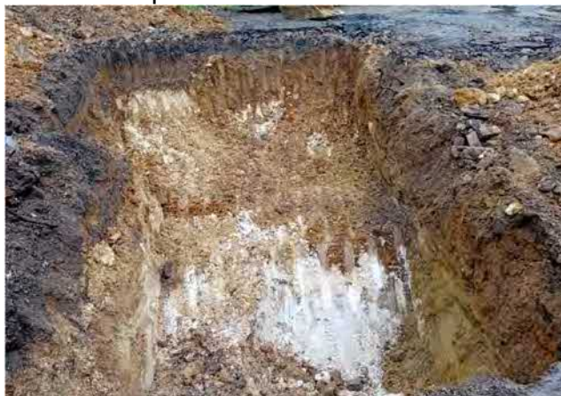
View of excavation
