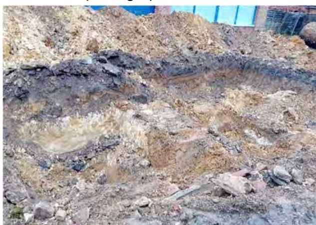
Excavation post tank removal
