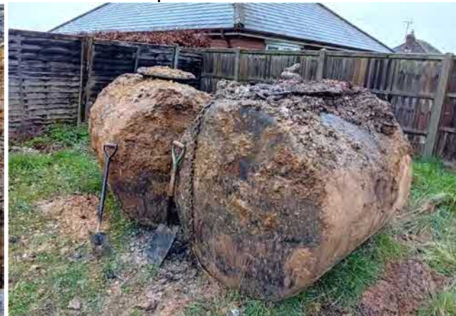
Two 500 gallon tanks removed
