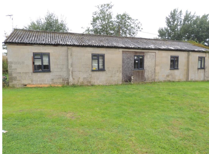
Photo 2: The eastern elevation
