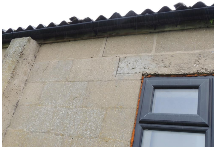
Photo 10: Typical section of eaves showing tight seal
