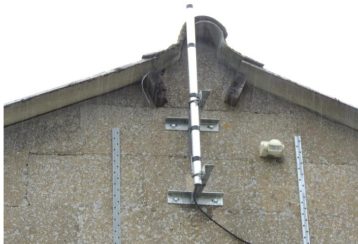
Photo 11: Showing tight seal to gable
