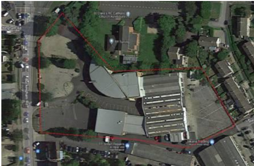
Figure 1: Site boundary of the land at Aylesbury (Former Range Rover Dealership), Buckingham Way
