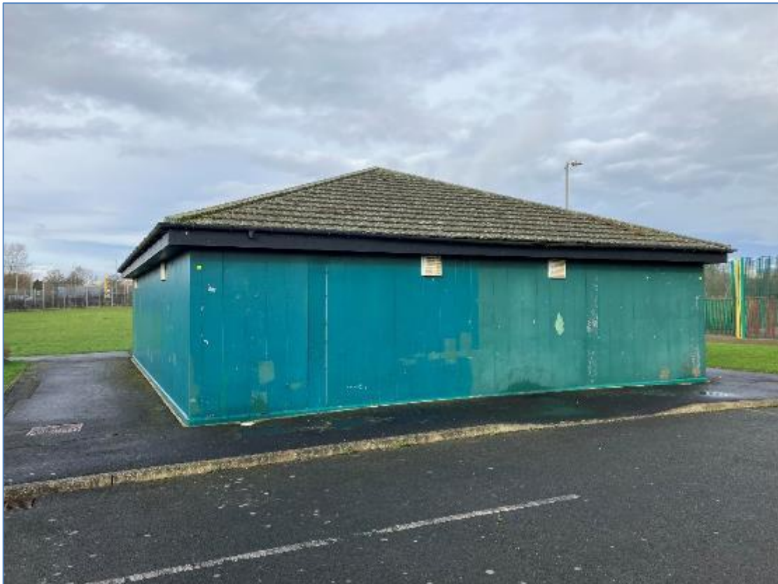
Photograph 4 – Building on Charlie Wayman Fields
