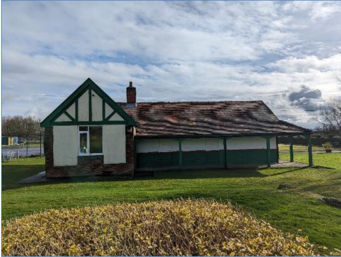
Photograph 5 – Building on Miners Welfare Ground
