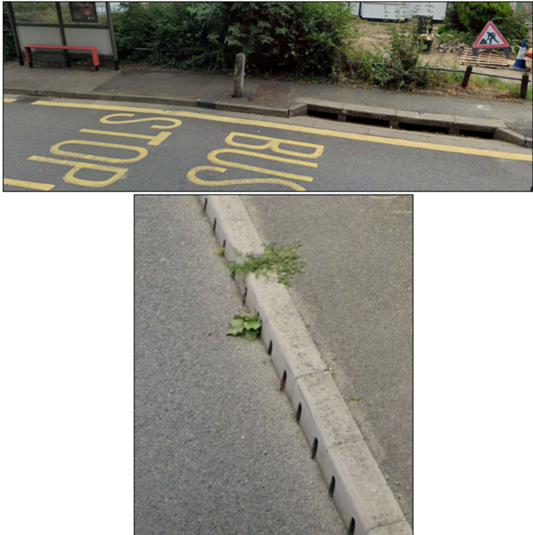
Figure 3.4 – Satellite imagery showing the drainage kerbs and highway drains along Rushmore Hill.
