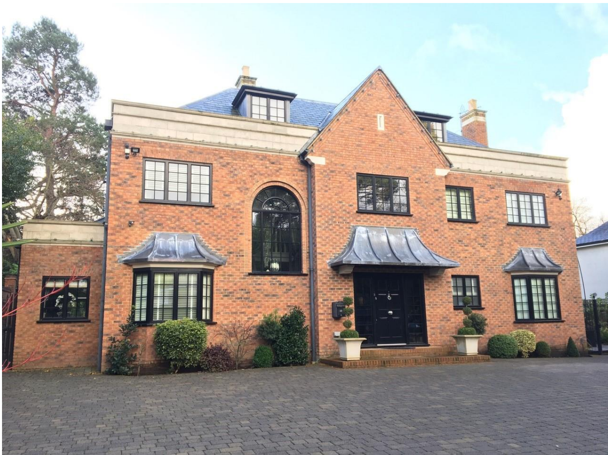
Fig.1 View of front of dwelling
