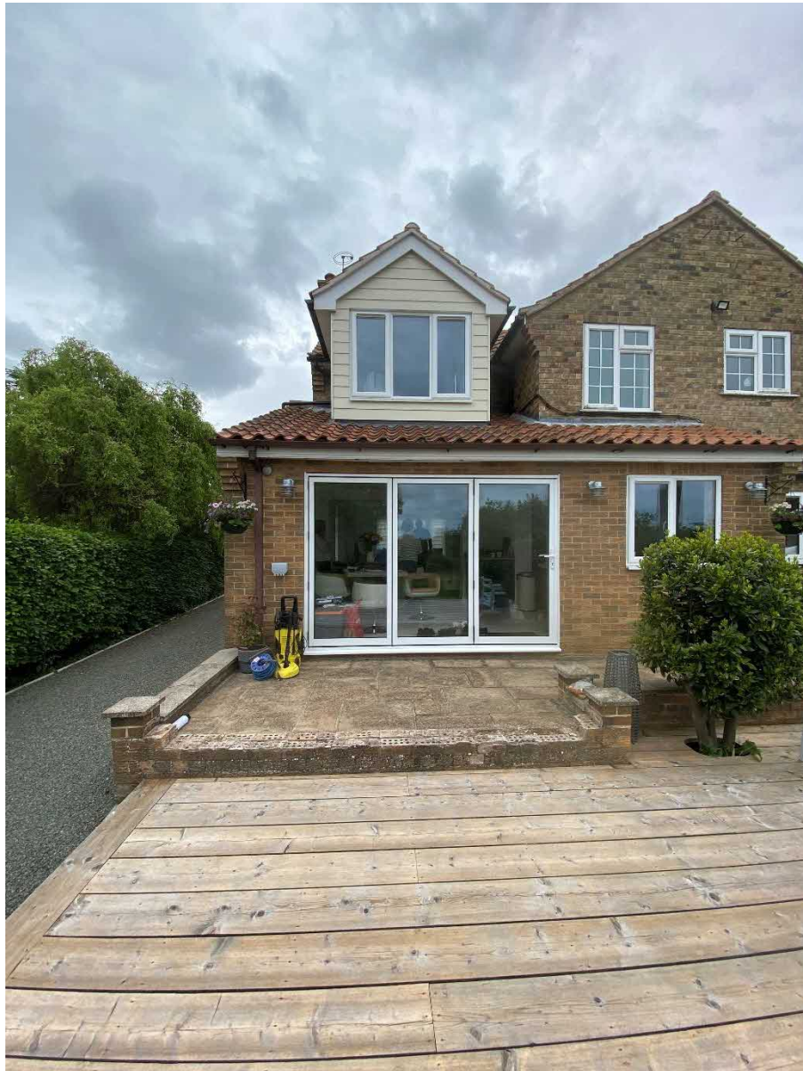
Existing Rear Extension.
