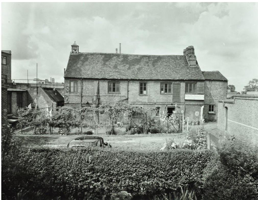
Figure 21: 1962 photograph of east elevation of the subject site. (LMA, 144584.)
