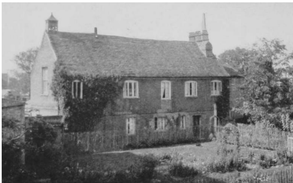
Figure 20: c. 1930 photograph of the east elevation of the subject site. (National Archives.)
