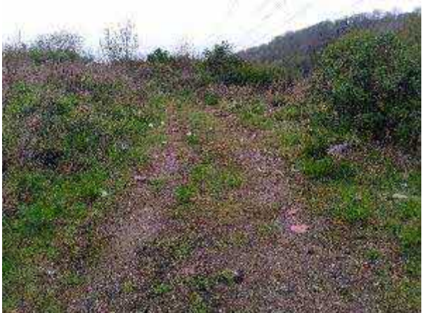
Steeply landfilled area of landfilled sparsely vegetated unsealed surface.
