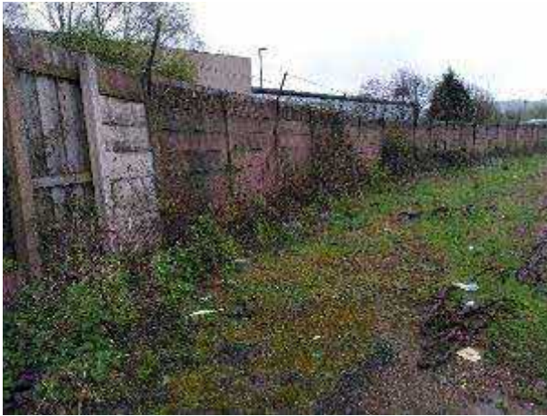
View of southern boundary concrete panel fence
