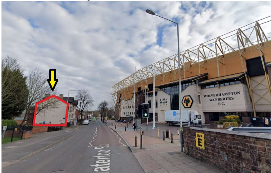
Figure 2 – Waterloo Road street scene
