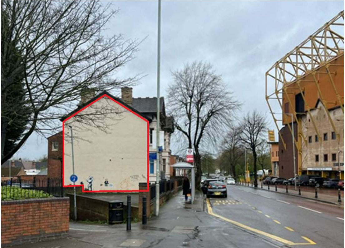
Figure 1 – The application wall (63 Waterloo Road)
