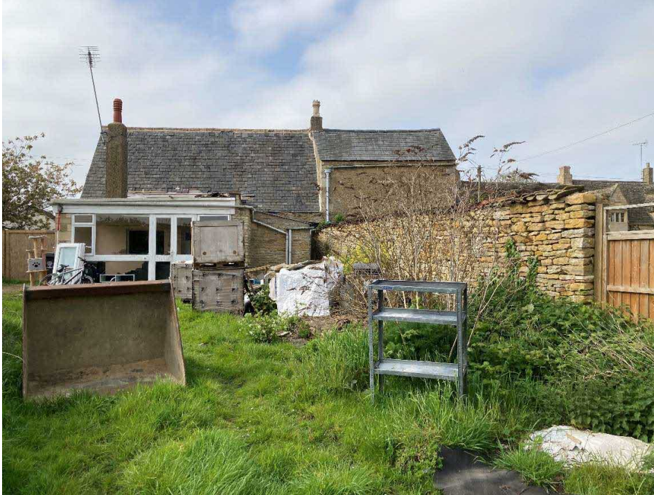
Figure 14. General view of rear. The slate roof covering on the rear of the 18 th -century cottage replaced Collywestons in the very recent past.
