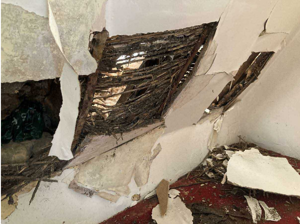
Figure 28. Detail of the reed backing.
