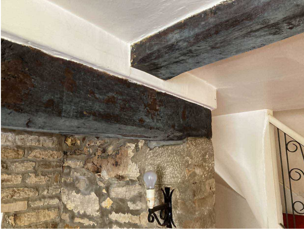
Figure 21. The chamfered beam above the bressumer. Neither may be original.
