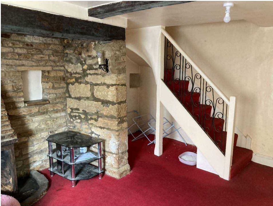
Figure 22. The staircase; probably 1970s but its upper part probably in original position.
