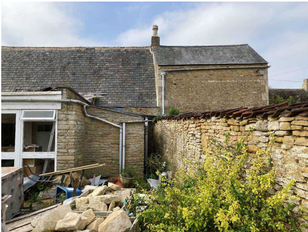
Figure 16. The rear extensions and boundary wall.
