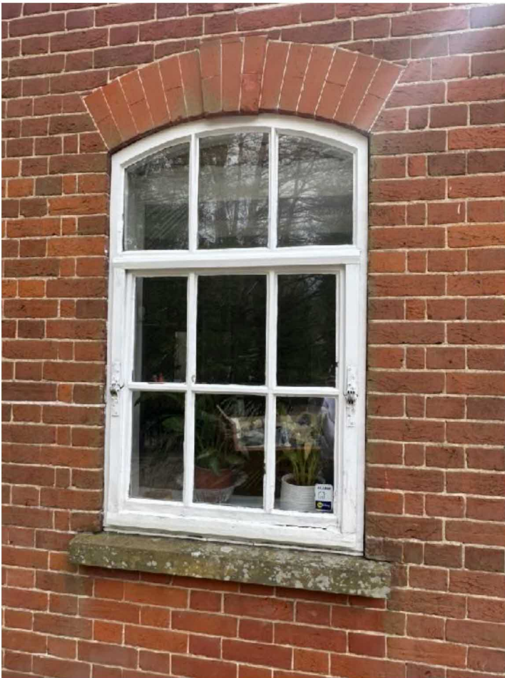
Plate 4: general view of window
