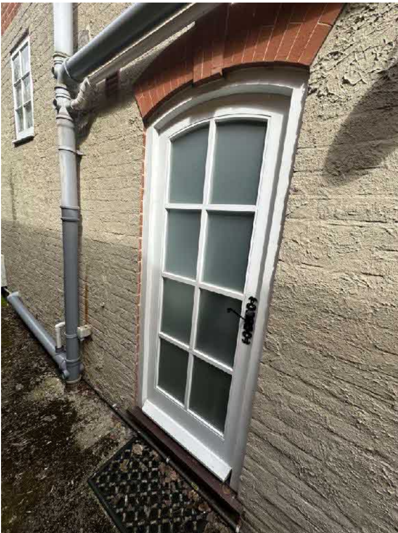
Plate 6: Existing side / side west elevation door
