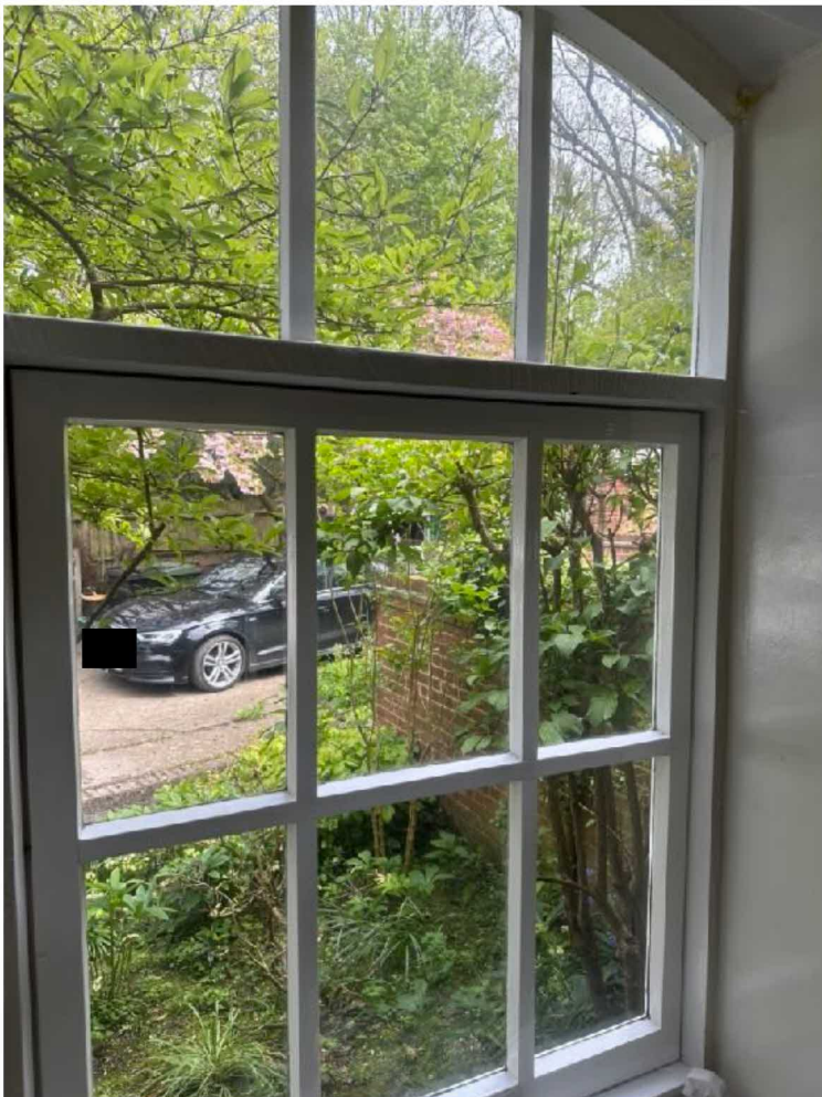
Plate 5: View of internal parts of window. Large glazing bars.
