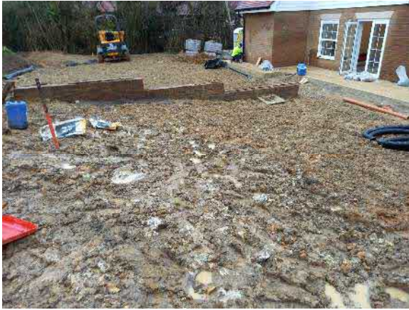
Plate 1 – Subsoil in rear garden of Plot 174 looking to 175, taken 13/12/2023.
