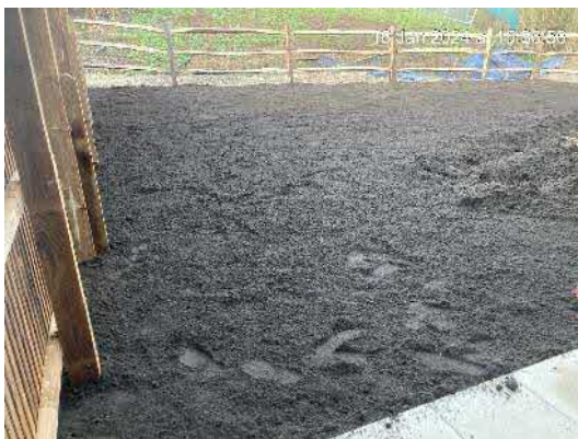
Plate 5 – Rear garden of plot 175 with topsoil placed. Taken by the client 16/01/2024.
