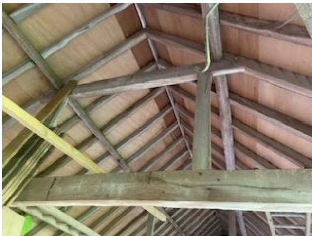
Typical roof arrangement of Barn 1
