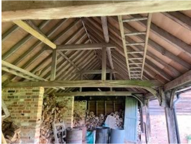
brick work piers in Barn 1
