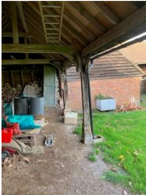
Timber posts with knee bracing, barn 1
