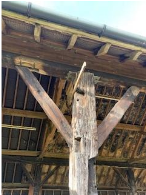
Barn 2 timber post with knee bracing.
