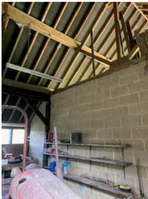
Existing blockwork wall in barn 2.
