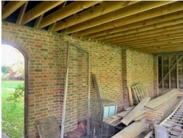
Masonry rear wall.
