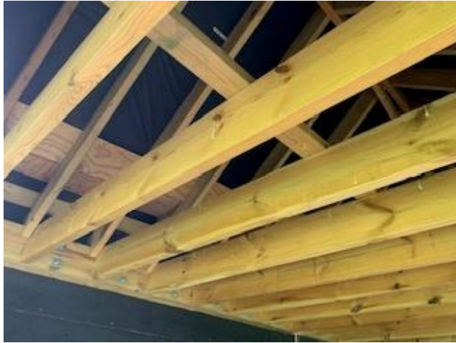
Roof timbers to barn 3
