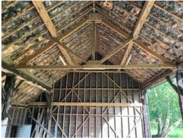
Typical timber arrangement in
