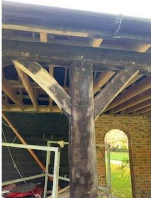
Barn 3 post and knee bracing detail.
