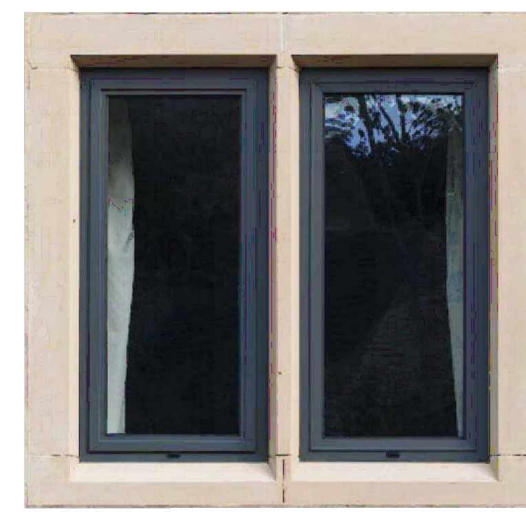
Painted window, Stone cill and surround
