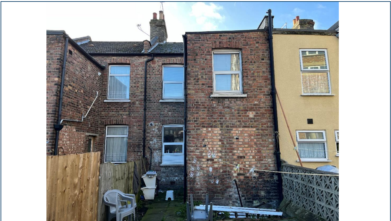
Photo 02 – Existing Rear Elevation
