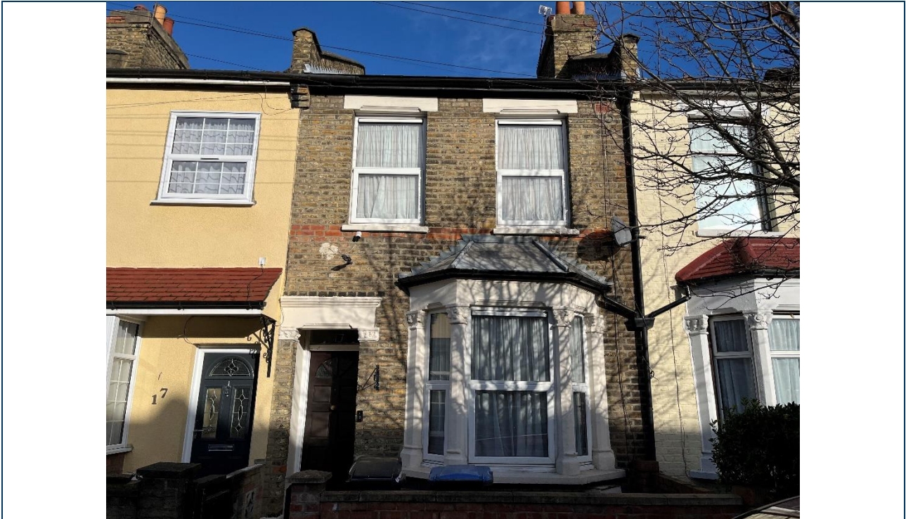
Photo 01 – Existing Front Elevation
