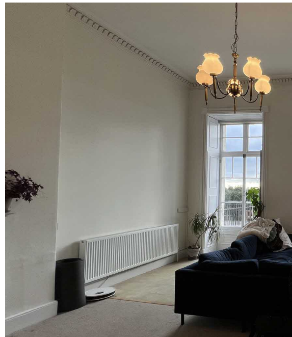
Existing sitting room radiator to be relocated
