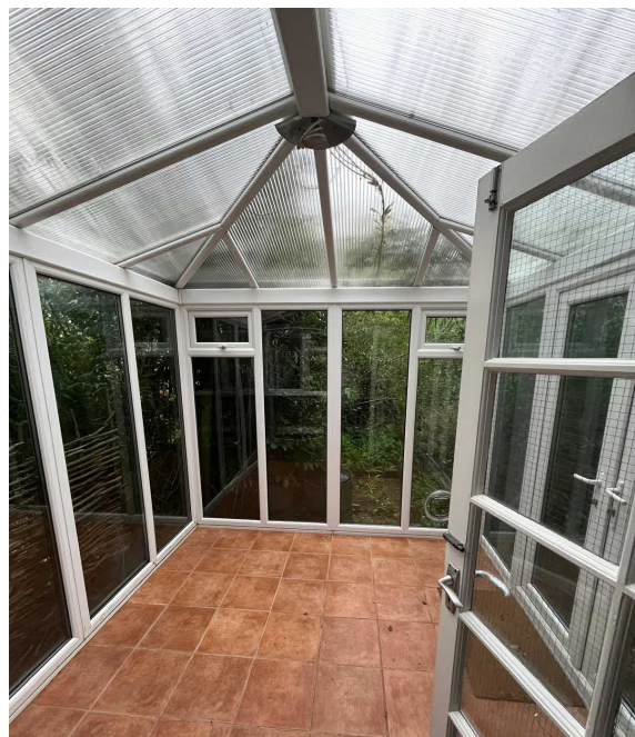
Existing white uPVC conservatory - poor quality of space internally.
