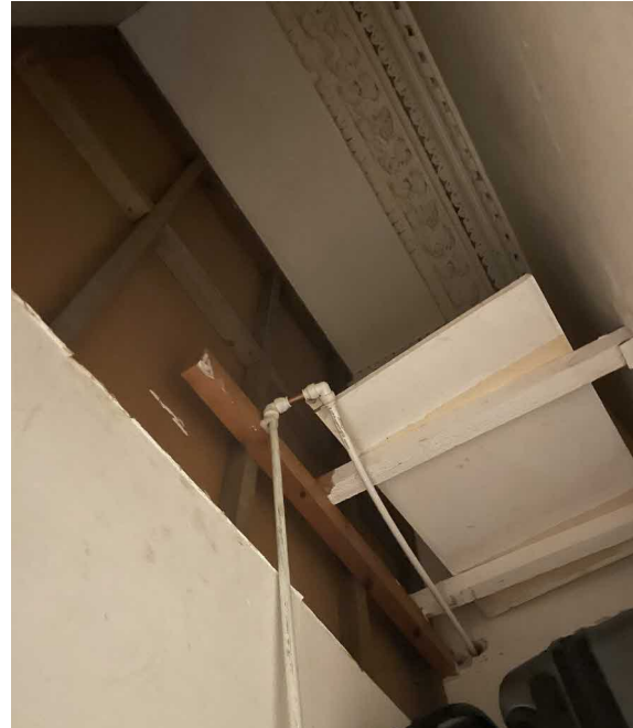
Original sitting room cornice in existing store room cupboard
