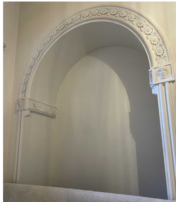
Original arched alcove in bedroom 1
