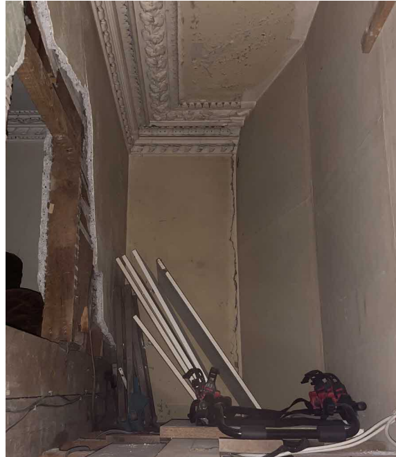
Original cornice above existing hallway
