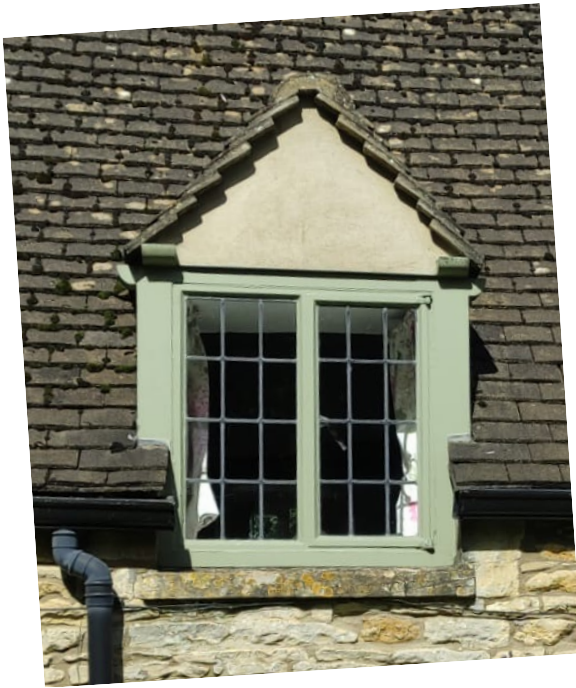
Timber subframe; Steel casement; single glazed with integrated lead
