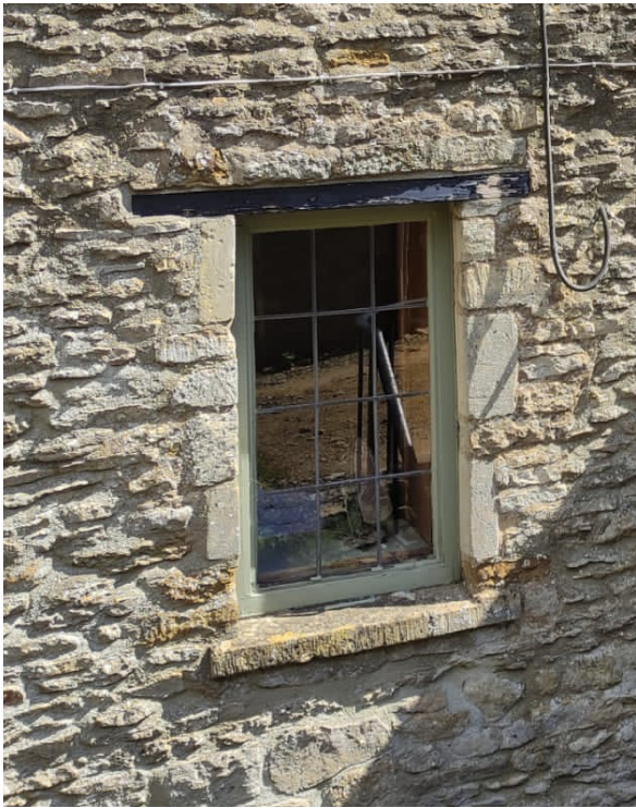
Timber frame; single glazed with stick on lead
