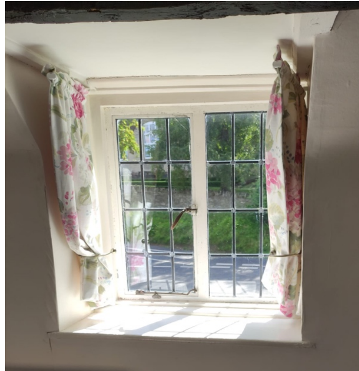
Timber subframe; Steel casement; single glazed with integrated lead
