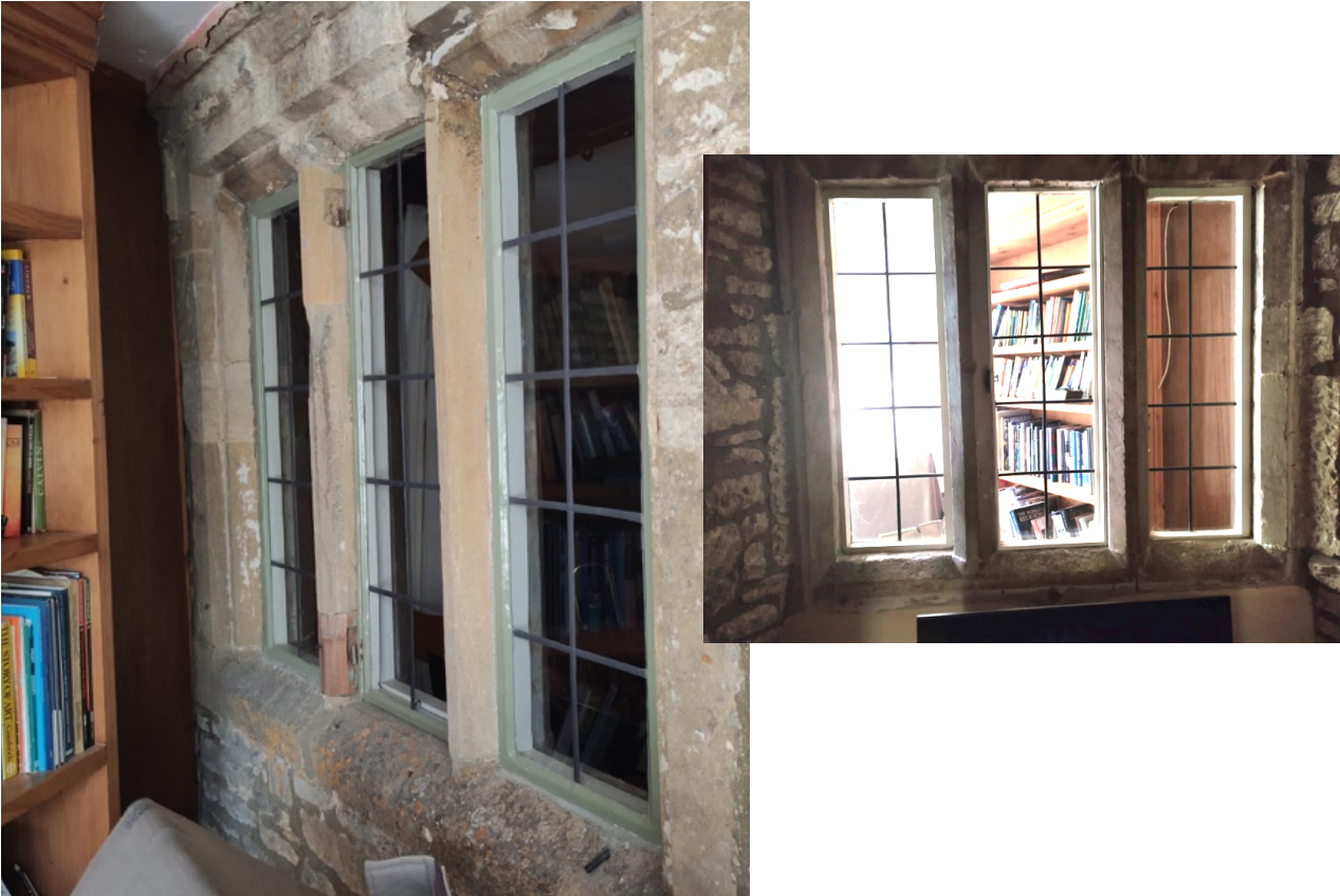
Timber frames, single glazed with stick on lead
