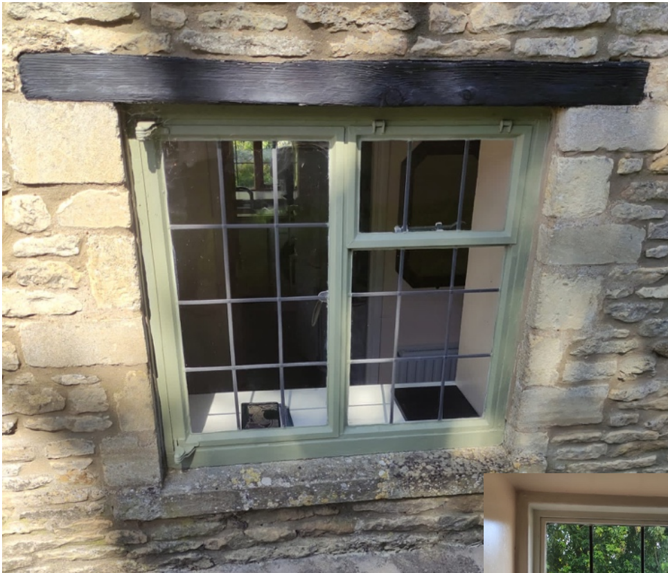
Timber subframe; steel casement; stick on lead; single glazed
