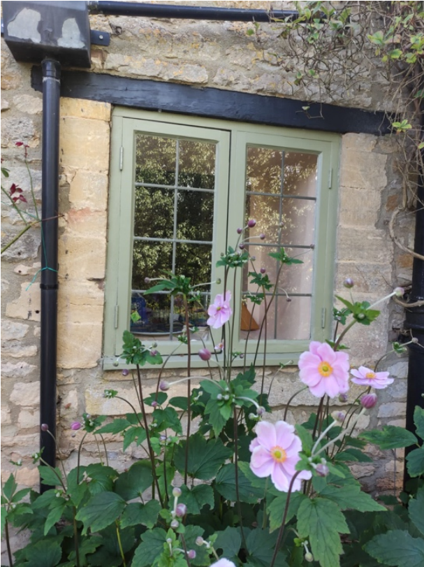
Timber frame & sill; single glazed with stick on lead
