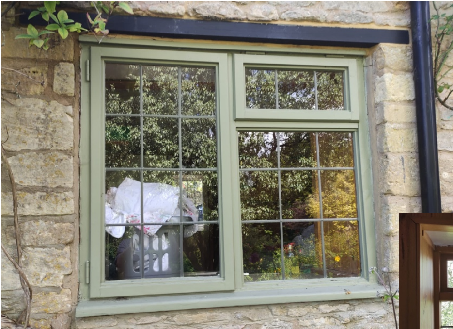
Timber frame & sill; single glazed with stick on lead
