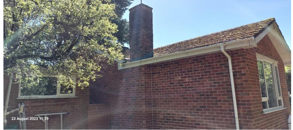
Photo 6: Northern elevation and external chimney of the bungalow.
