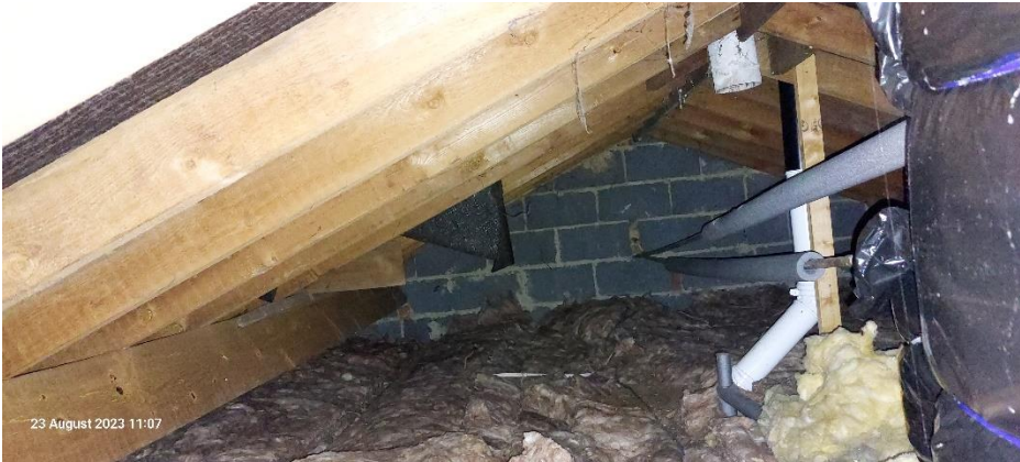
Photo 1: Internal loft void of bungalow.
