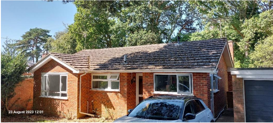
Photo 4: Front elevation of the bungalow.
