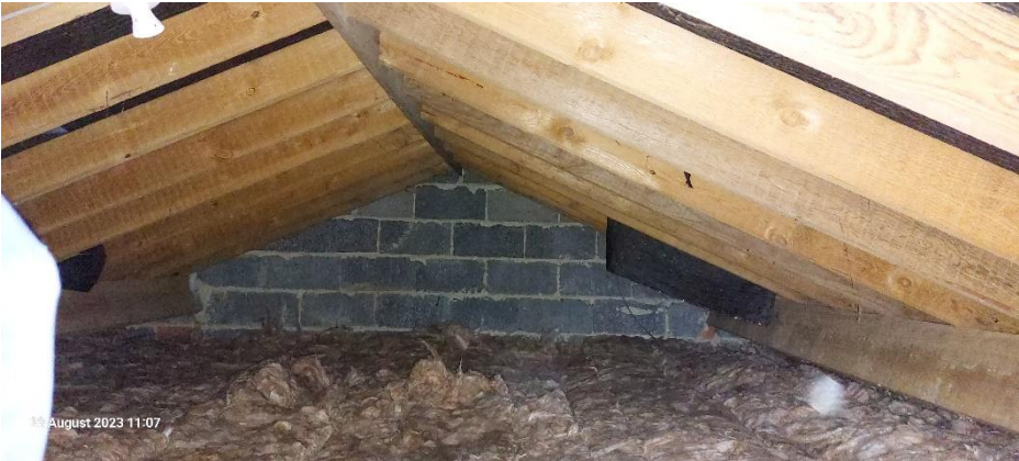
Photo 2: Internal loft void of bungalow.
