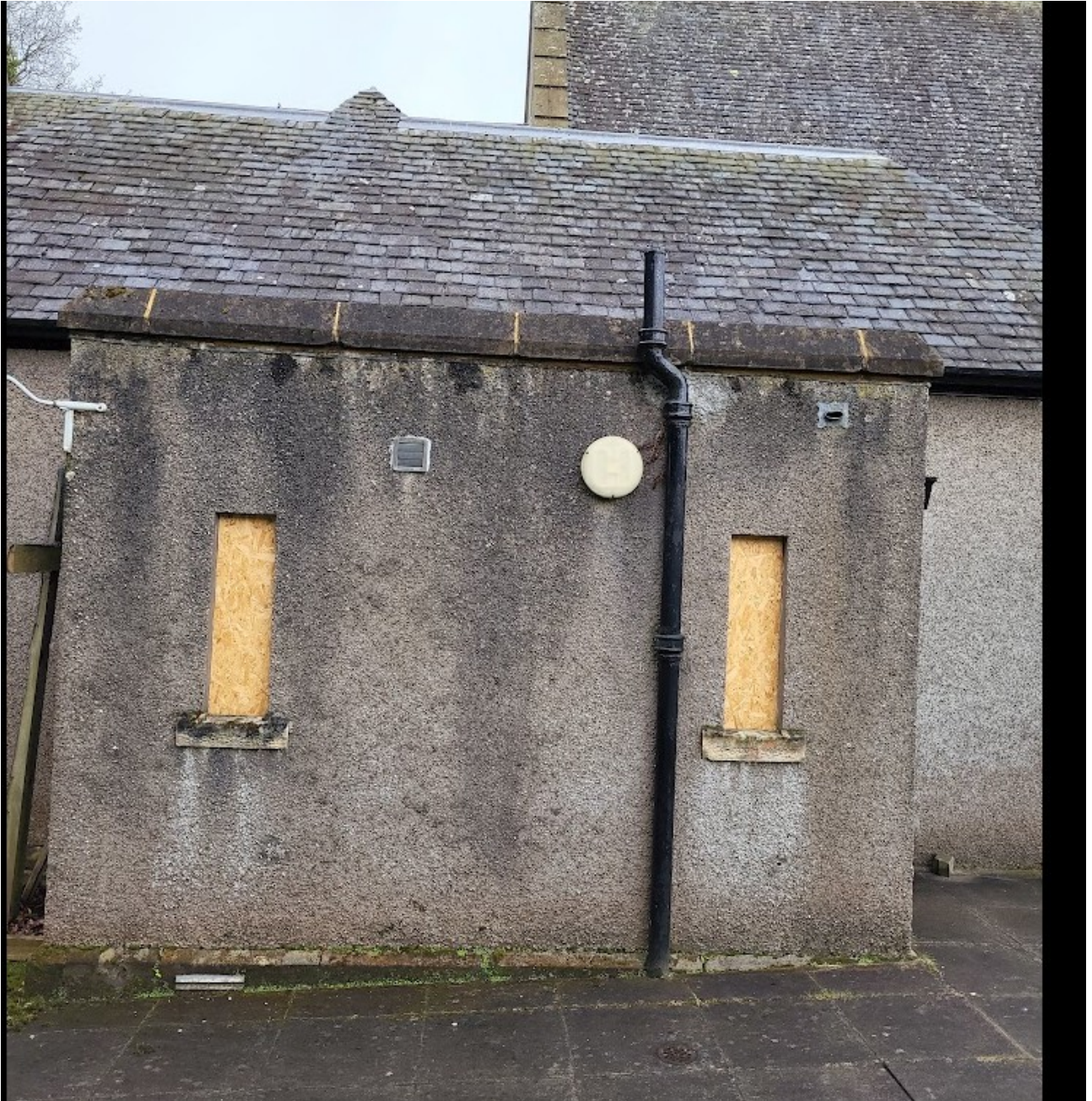
EXISTING VESTRY VESTIBLE WINDOWS
