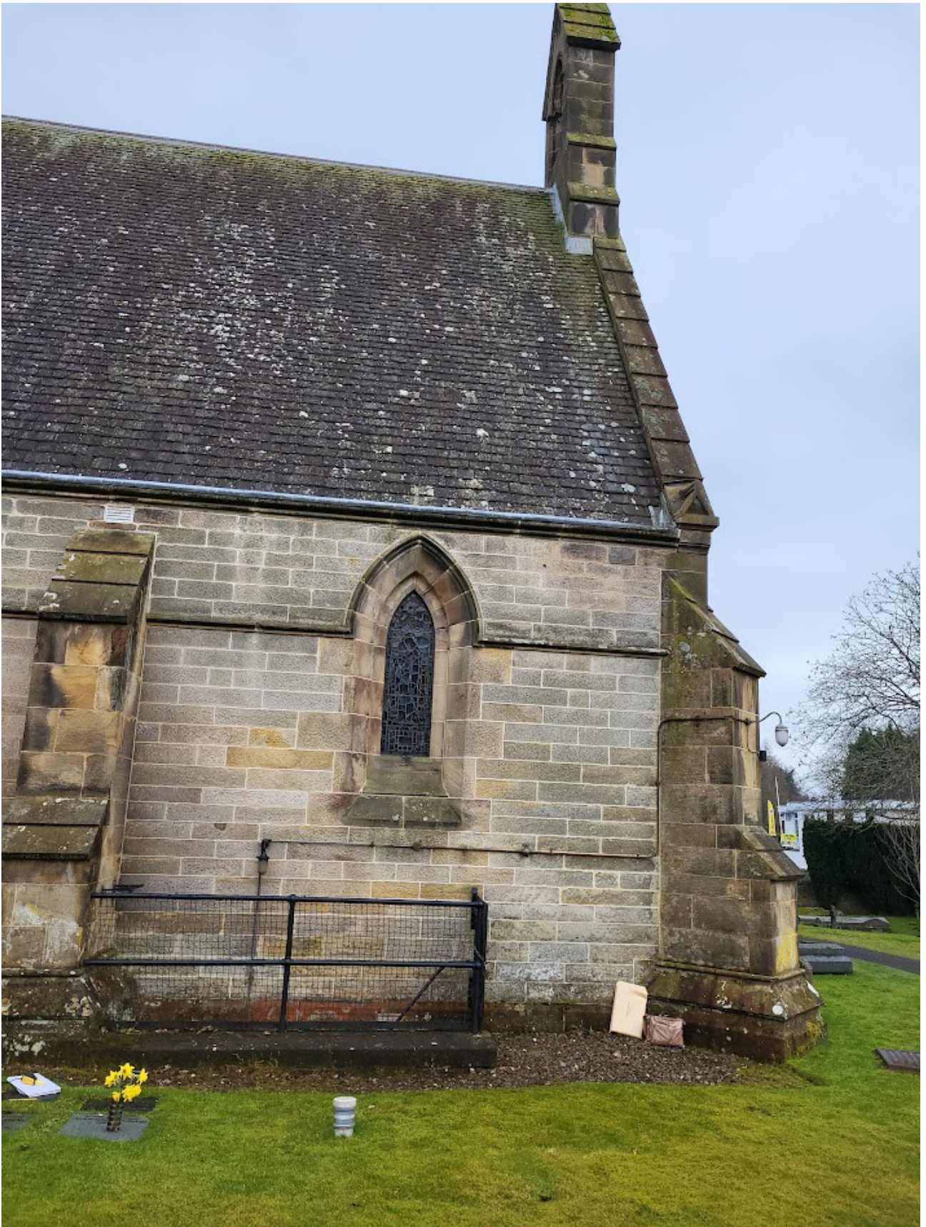
EXISTING RAILINGS AT ACCESS TO BASEMET
