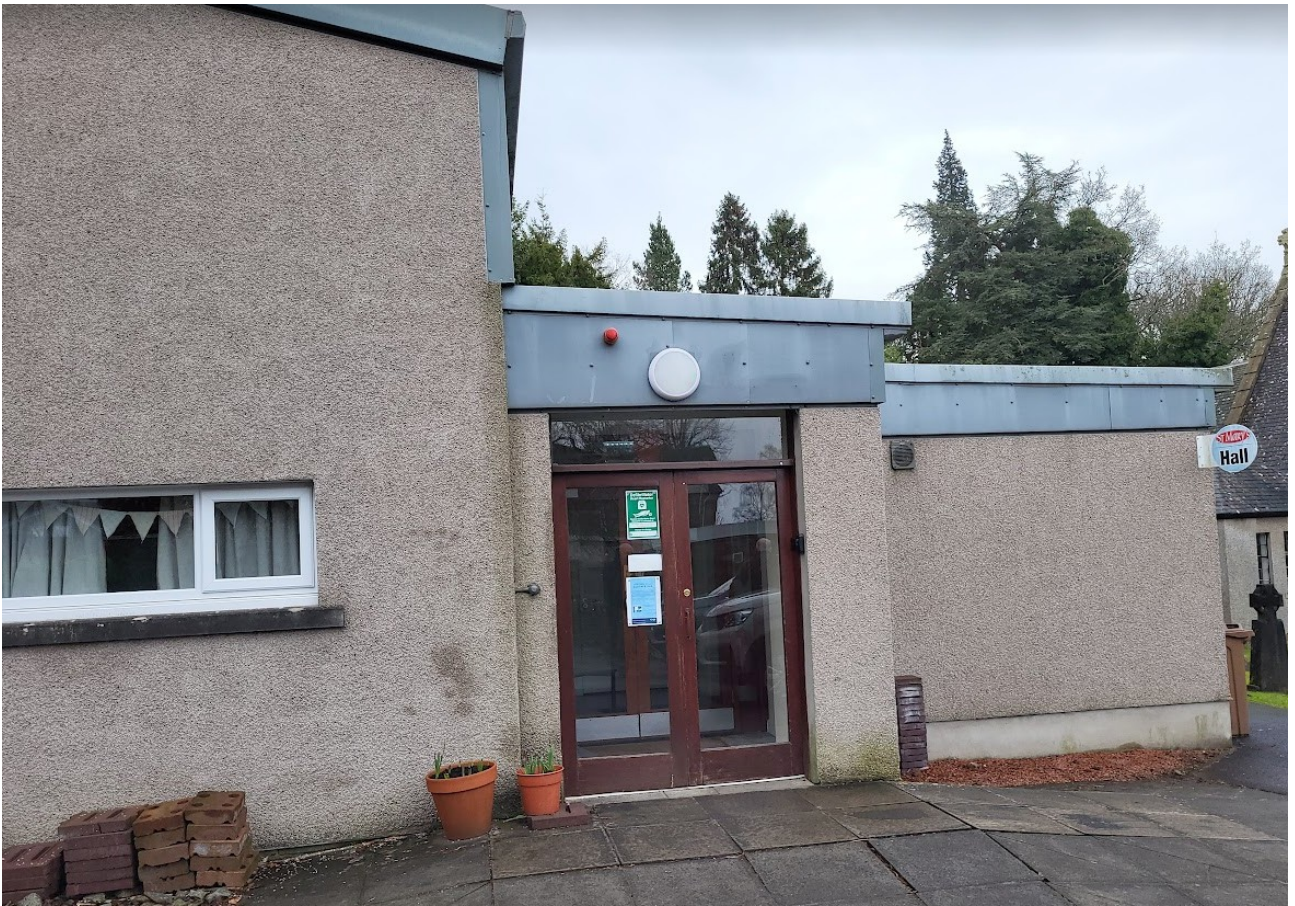
EXISTING ACCESS DOOR TO HALL
