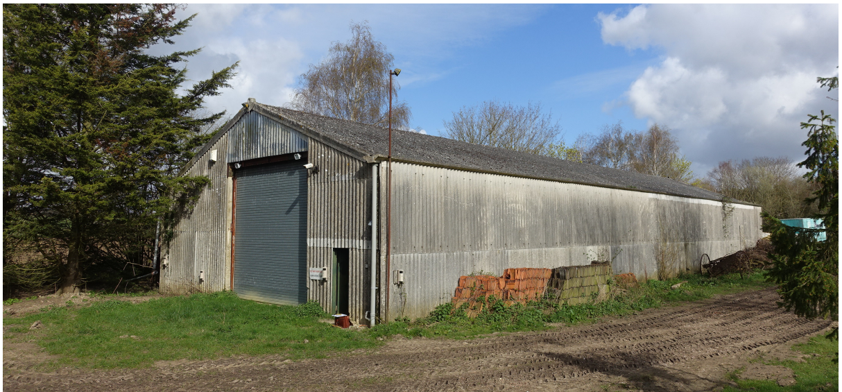
Picture 3 – south end of barn
