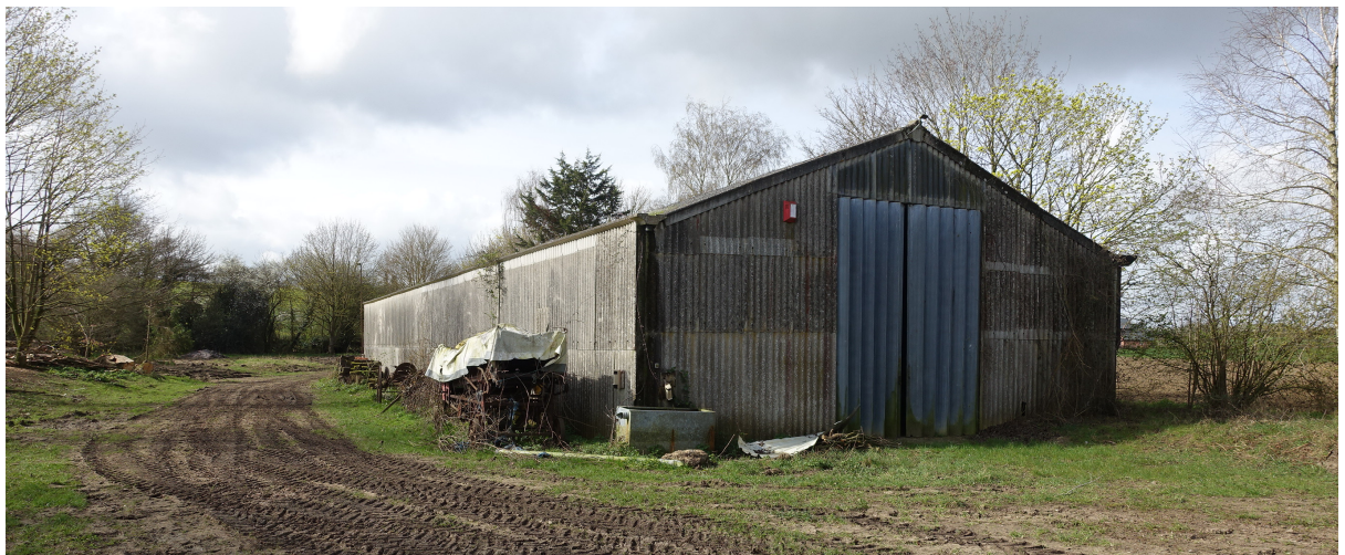
Picture 4 – north end of barn
