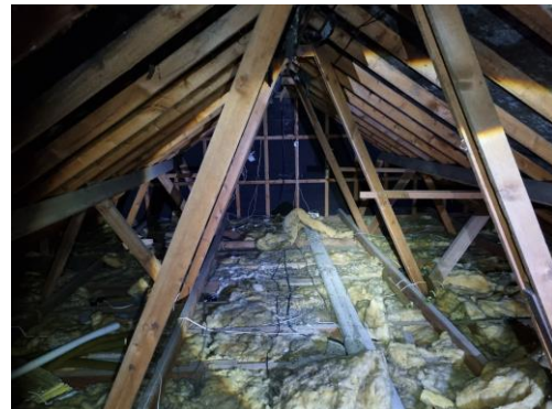
Figure 4.12. Loft space of Building 1
