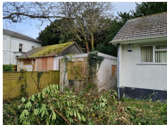
Figure 4.16. Southern and eastern elevations of Building 4
