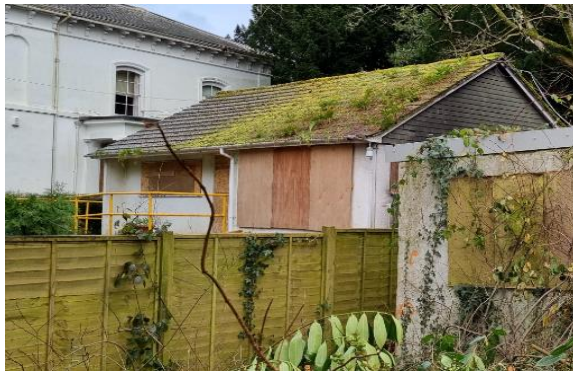
Figure 4.11 South-eastern elevation of Building 1
