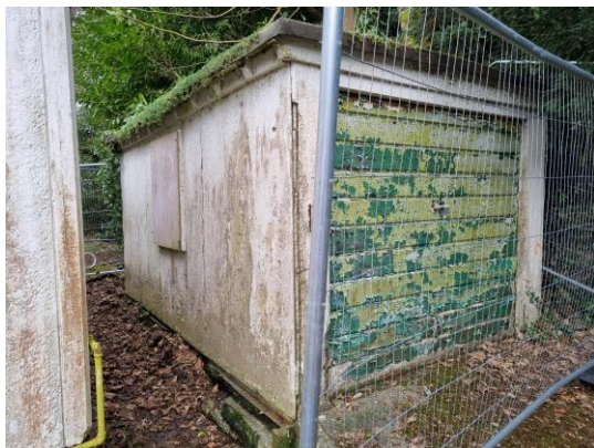
Figure 4.15. Southern and eastern elevations of Building 3
