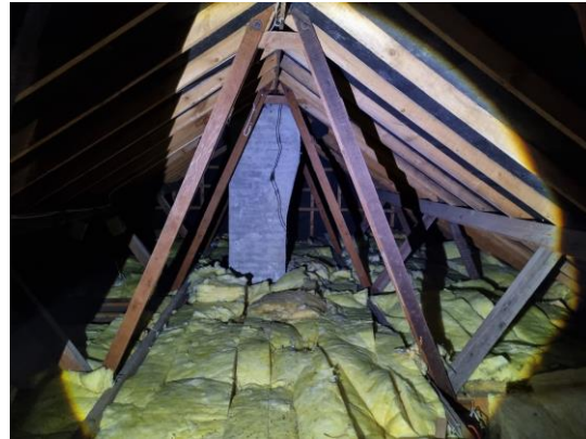
Figure 4.14. Loft space of Building 2
