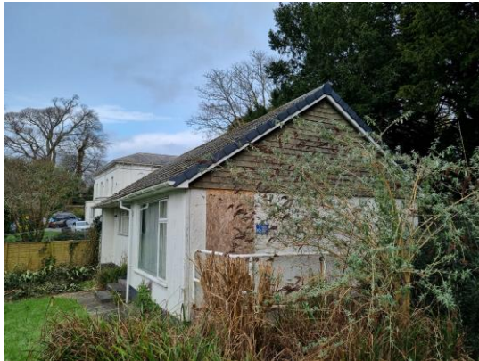
Figure 4.13. South and eastern elevations of Building 2
