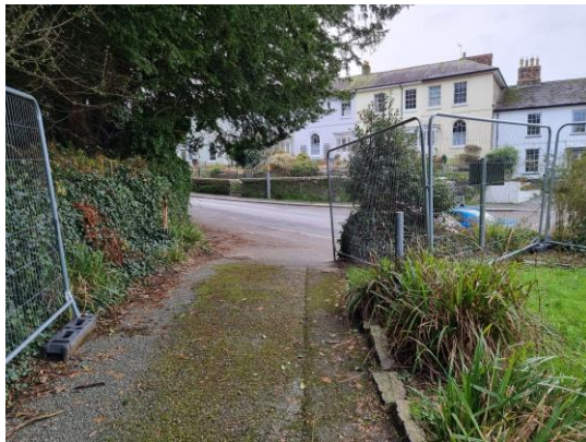
Figure 4.3 Tarmac road within the south-eastern extent.
