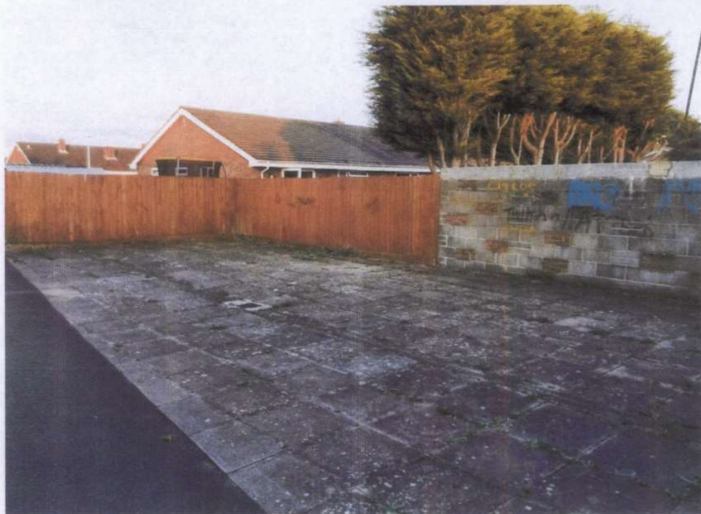
Photo #3: Photo of existing boundary with 1 Plover close (Concrete block wall) and boundary with 2 Cormorant close (wooden fence) Only the Concrete block wall boundary would be removed under this proposal, our neighbour's fence would remain.
