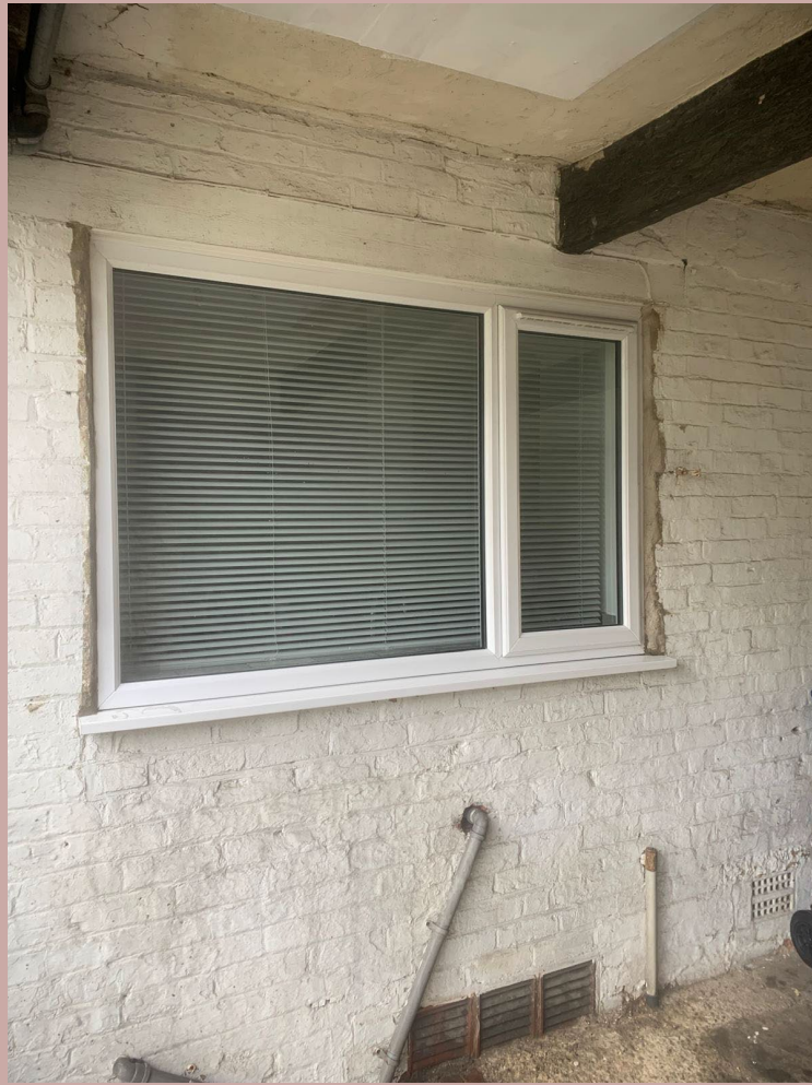
Rear ground floor window replaced with like-for-like UPVC
