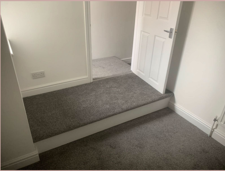
Raised floor for soil pipe
