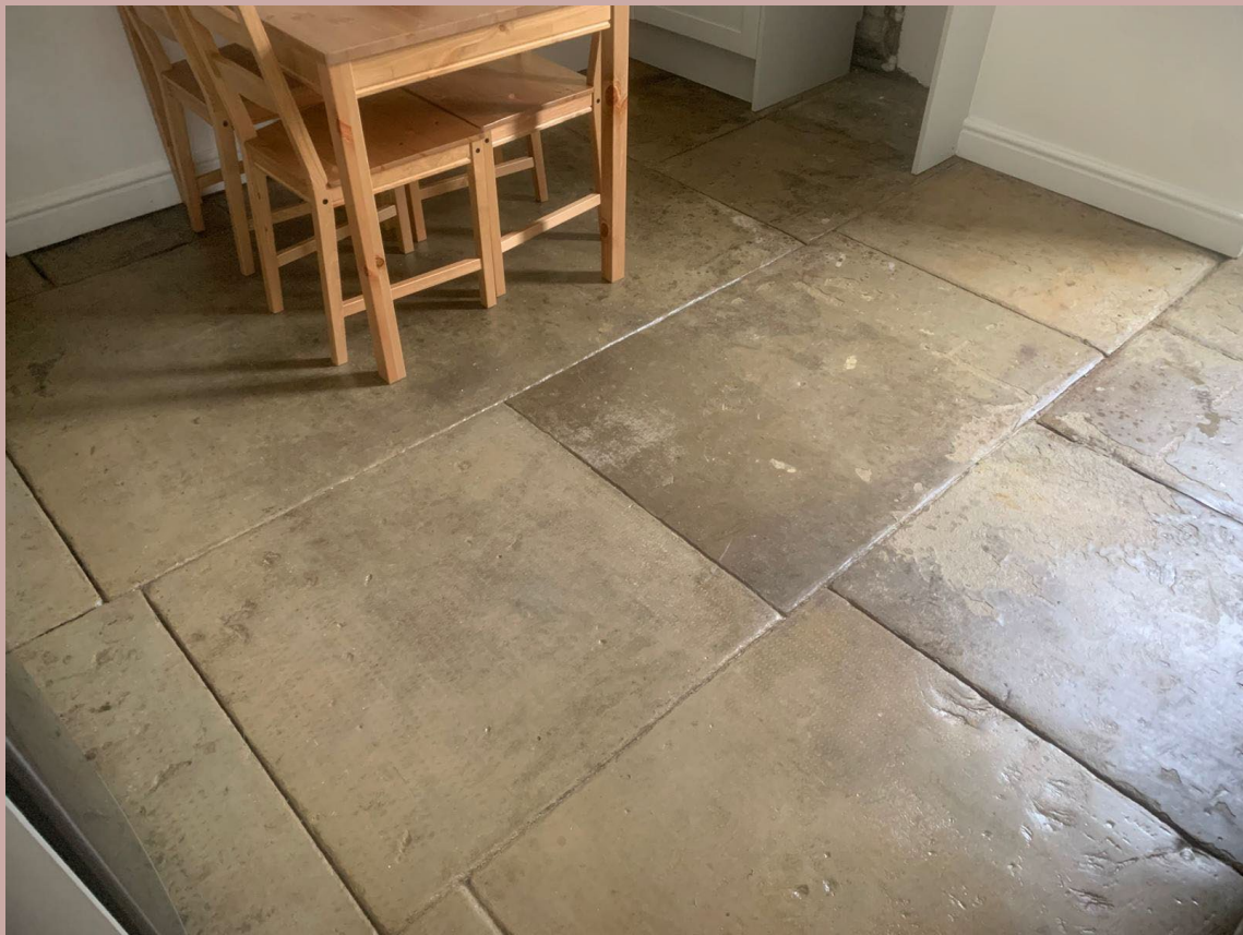
Kitchen stone floor restored
