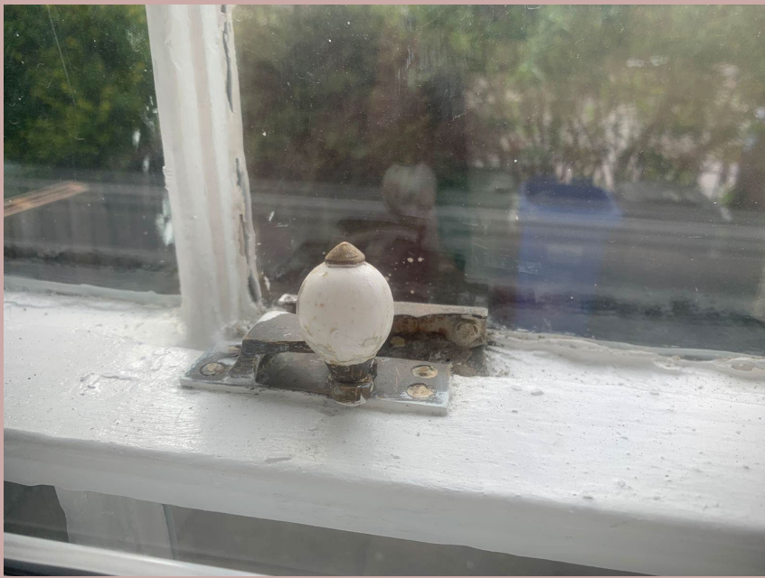
Original fittings to sash windows retained
