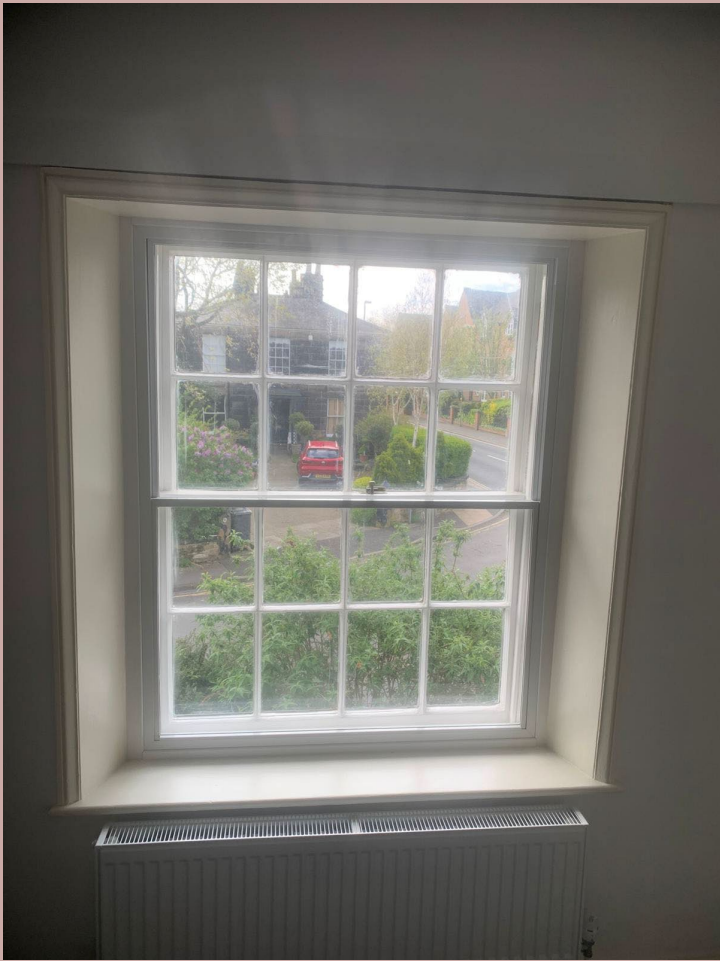
Front facing bedroom window (internal)
