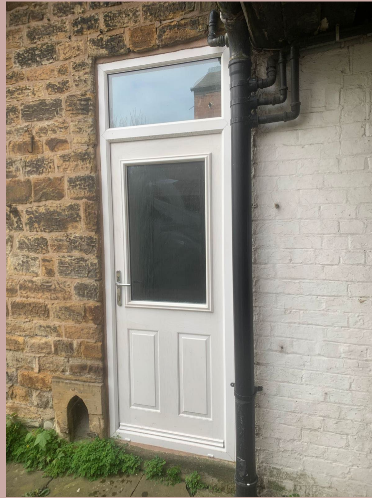
Rear door replaced with like-for-like UPVC
