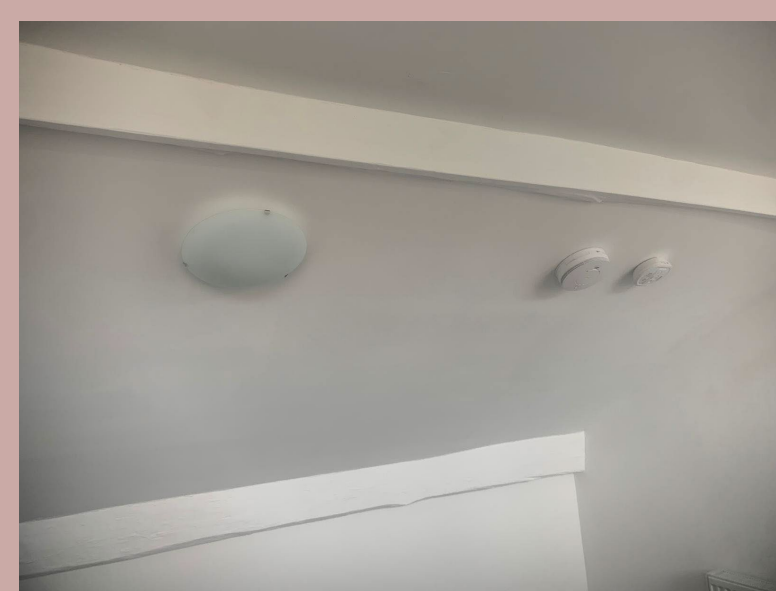
Second floor beams
