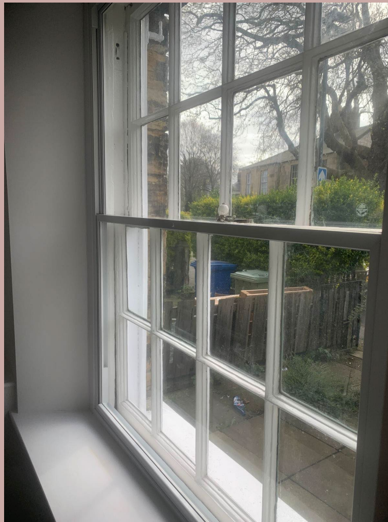
Secondary Glazing in Ground Floor Sash Window
