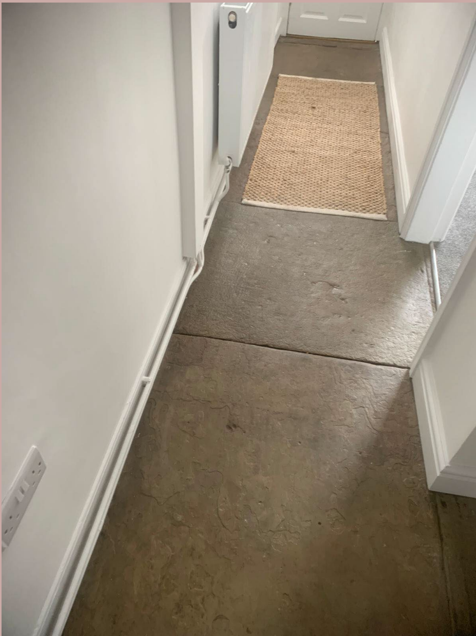
Hallway restored stone floor
