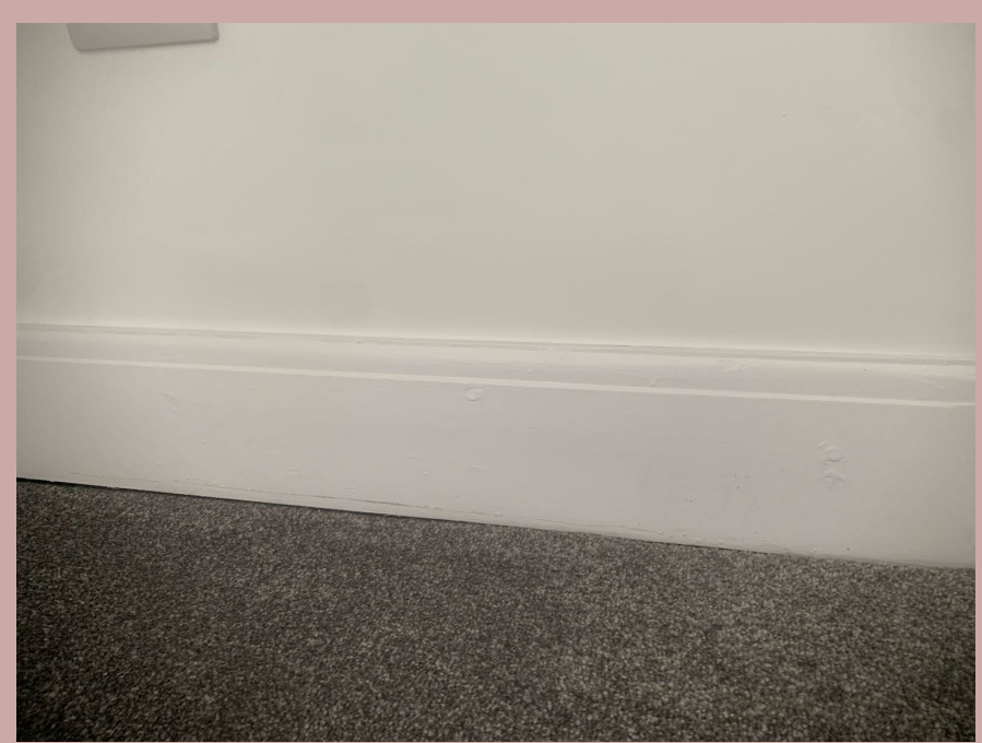
Second floor skirting
