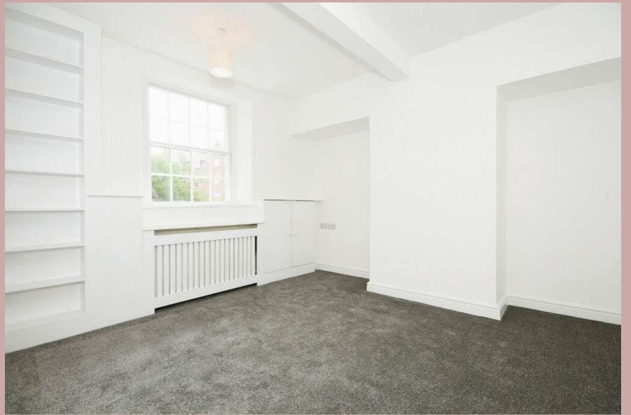
Living room afterwards (covered fireplace)
