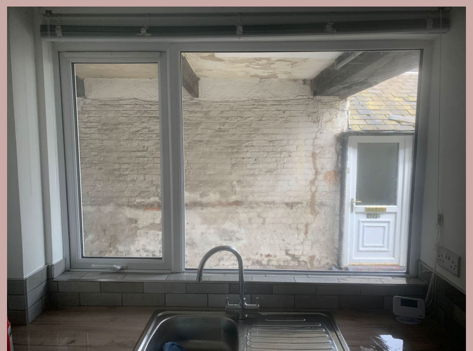
Kitchen window (internal)
