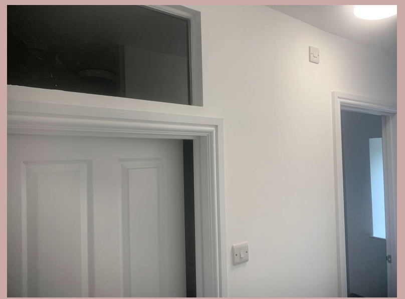
Stud wall replacing unsafe block wall
