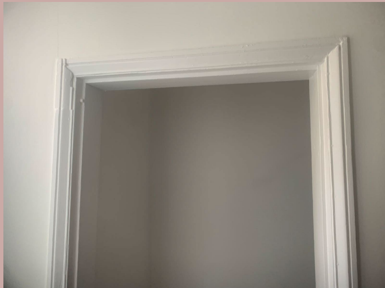
Kitchen to stairs door frame
