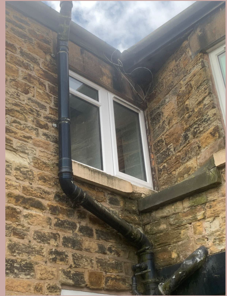
Rear first-floor window replaced with like-for-like UPVC
