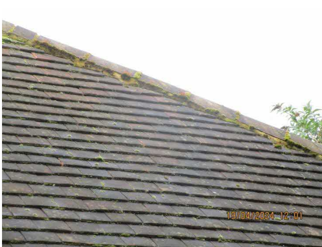
Photos 5 and 6 – Hip and ridge tiles are tightly fitted. The roof tiles are tightly fitted (apart from three gaps under tiles in areas which are completely unaffected by the proposals) such as the one shown in the red box below.
