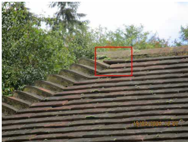
Photos 5 and 6 – Hip and ridge tiles are tightly fitted. The roof tiles are tightly fitted (apart from three gaps under tiles in areas which are completely unaffected by the proposals) such as the one shown in the red box below.
