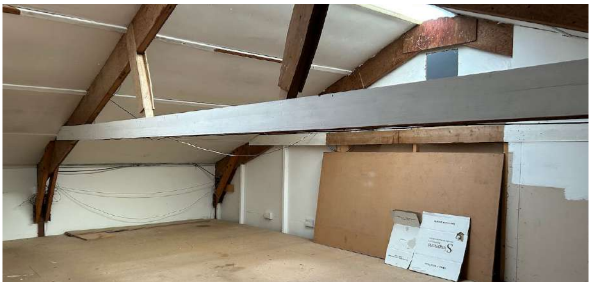
Photograph 9. Second storey section of Building 2
