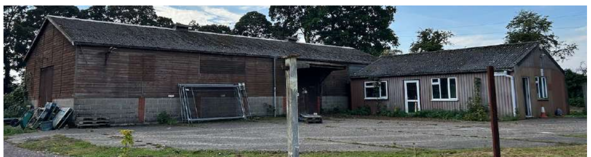
Photograph 5. Buildings 1 (on the right) and 2 (on the left) – north aspect
