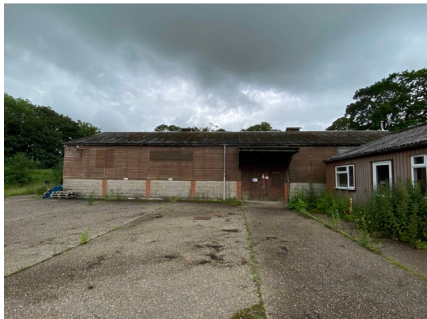
Both structures viewed from the site entrance
