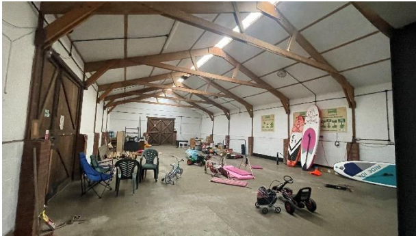
Photograph 8 Internal View of Building B
