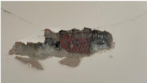
Photograph 2 Exposed Column in Wall of Building A
