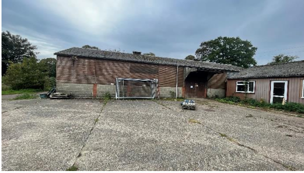
Photograph 7 North Elevation of Building B
