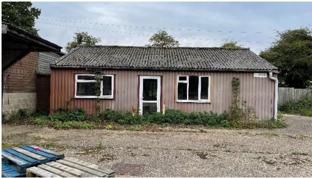
Photograph 1 East Elevation of Building A
