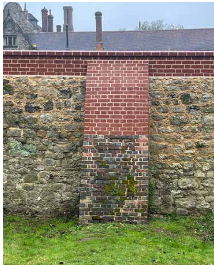
Figure 3.0.7 (below left): A buttress on the Laundry Courtyard wall, the upper section recently re-constructed. Note the lower original works entirely in traditional brickwork.
