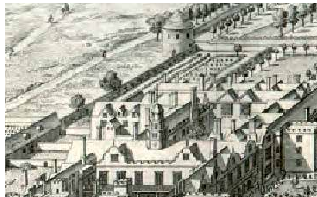
Figure 2.2.2 (right): A detail from the engraving above of the garden walls that pertain to this application (the round turret or dovecot has been lost).
