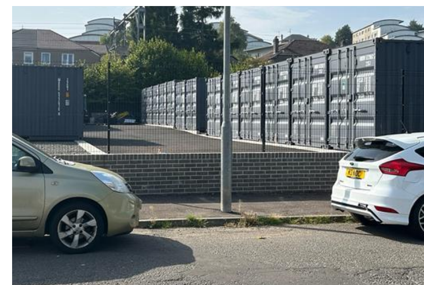
2M HIGH V-MESH PERIMETER FENCING PROPOSED. (WITH LOW BRICK RETAINING WALL, IF NEEDED). PERIMETER FENCING AROUND ALL BOUNDARIES.
