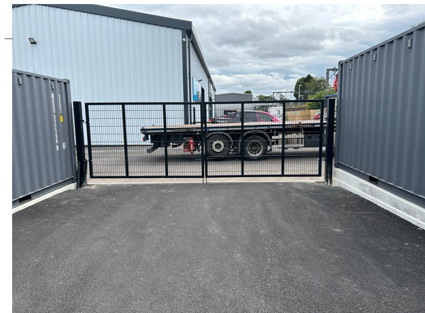
6M WIDE STEEL GATES TO VEHICLE ENTRANCE.
