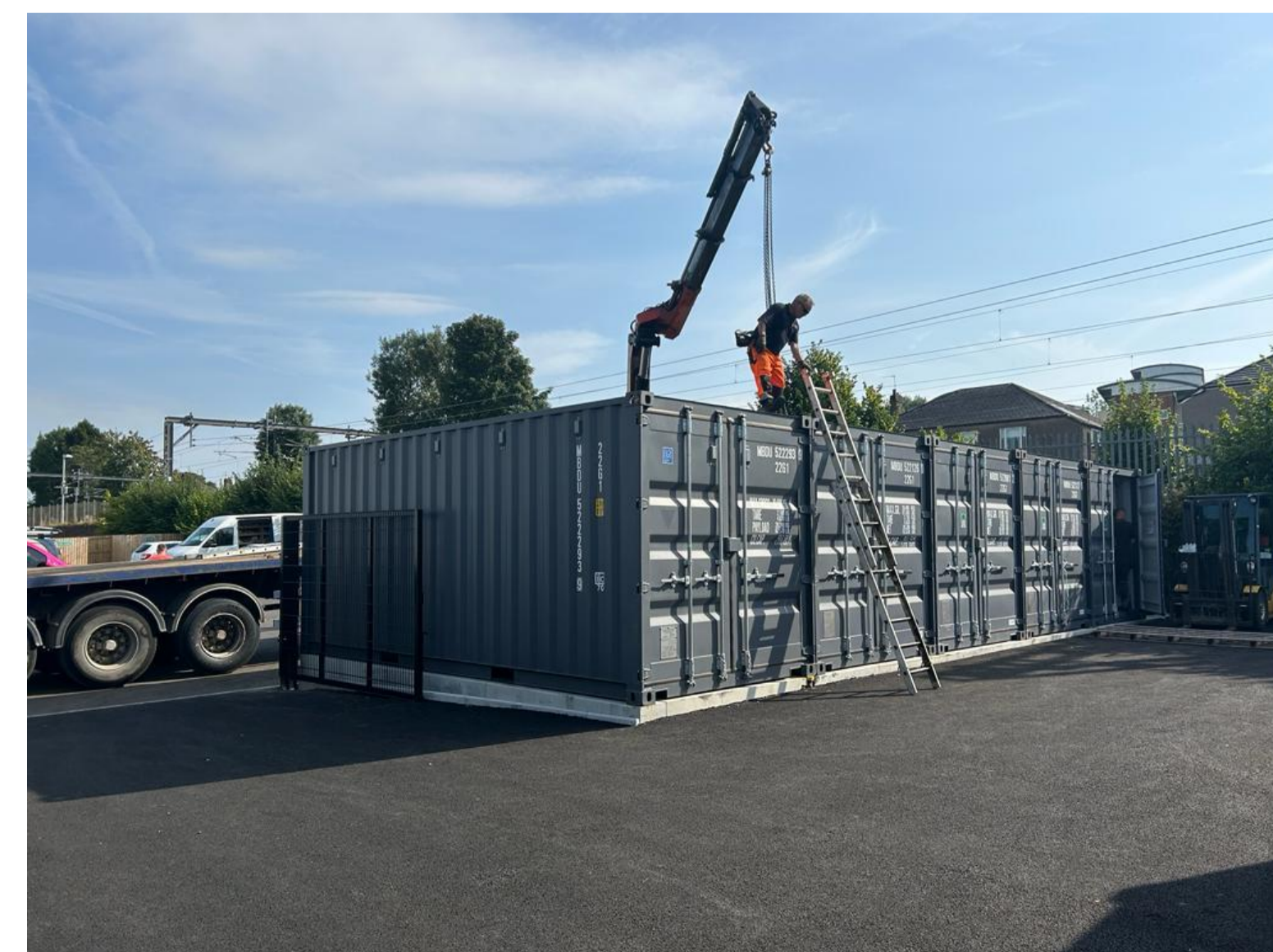
STANDARD 20FT SHIPPING CONTAINERS PROPOSED TO BE INSTALLED ONSITE FOR LETTABLE STORAGE.
