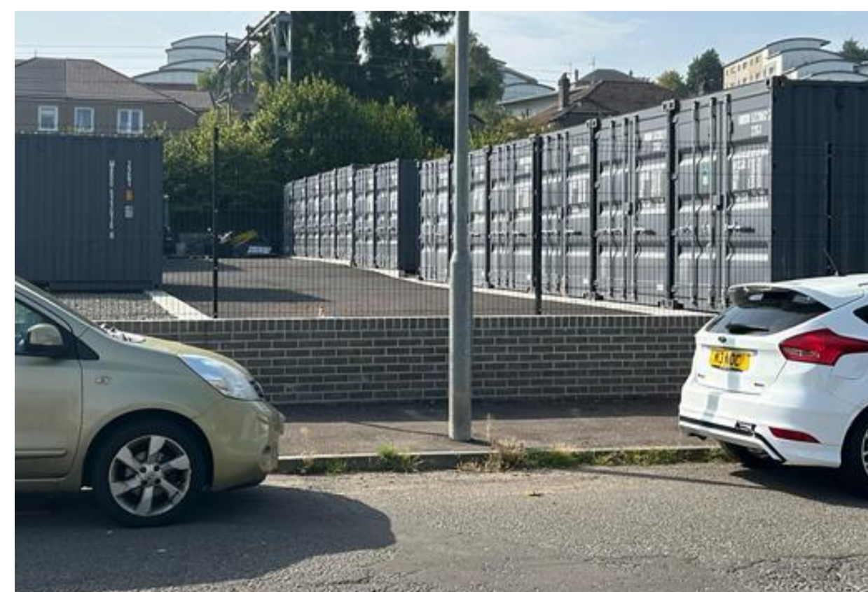
PHOTO ABOVE OF 2M HIGH V-MESH PERIMETER FENCING PROPOSED (WITH LOW BRICK RETAINING WALL). PERIMETER FENCING AROUND ALL BOUNDARIES.
