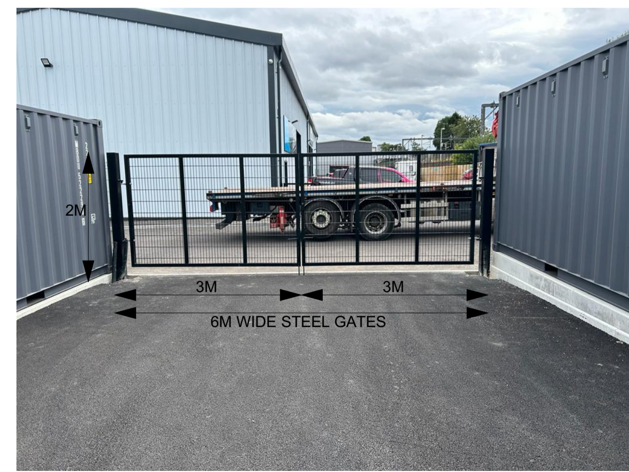
6M WIDE STEEL GATES TO VEHICLE ENTRANCE.
