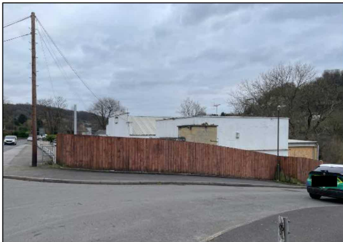
Plate 19: West elevation as viewed from junction between London Road and Arundell Mill Lane to the north-west.
