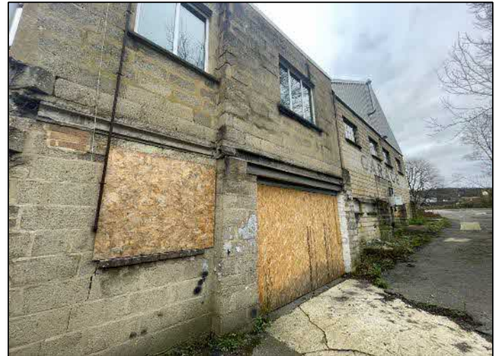
Plate 17: South elevation as viewed from the south-west.
