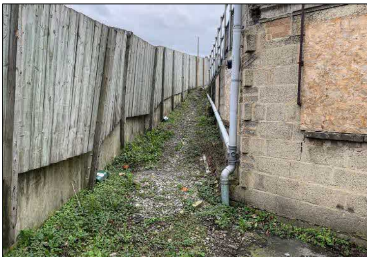
Plate 27: View looking north-east along western boundary of plot.
