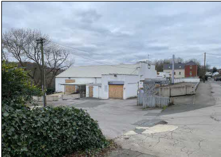
Plate 15: East elevation as viewed from the south-east.
