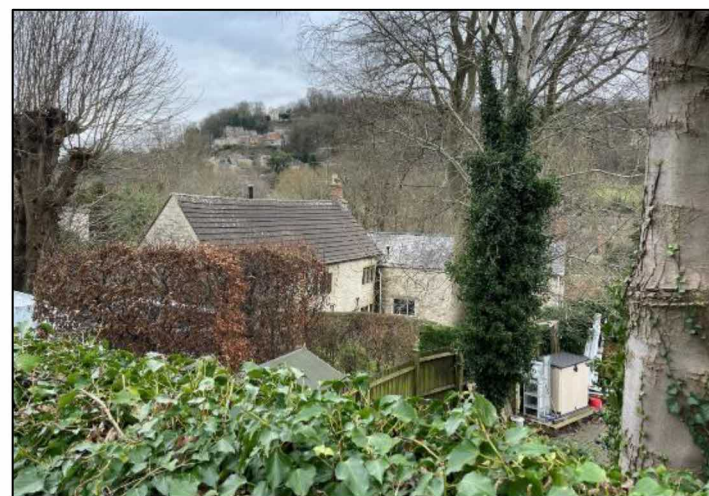
Plate 46: Mill house at Arundell Mill as viewed from London Road to the north-east.
