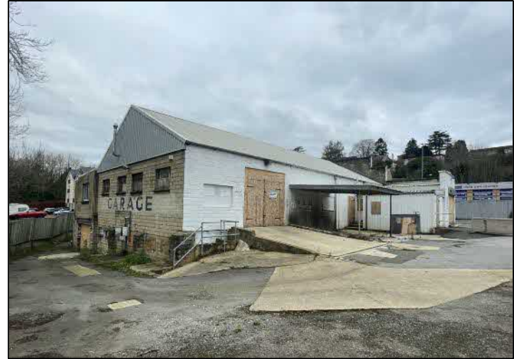
Plate 16: East (right) and south (left) elevations as viewed from the south.
