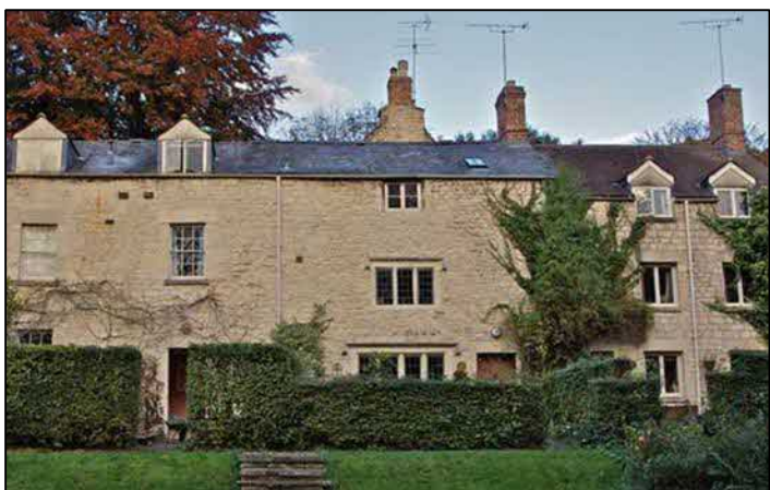
Plate 32: Mill house at Arundell Mill as viewed from the south. 18
