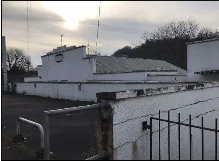
Plate 14: Principal north elevation as viewed from the north.
