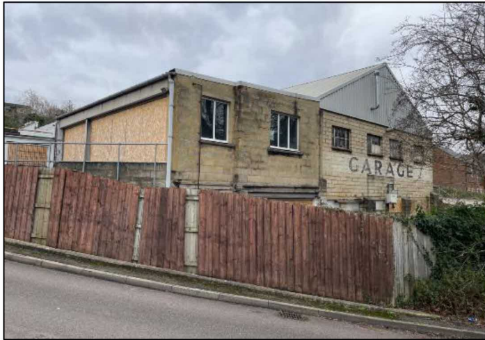
Plate 18: South elevation as viewed from Arundell Mill Lane to the south-west.
