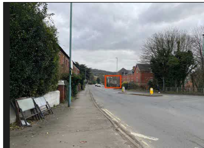
Plate 42: View looking south-east along London Road towards Site from section of Conservation Area to the north of Lower Dorrington Terrace, with heavily glimpsed visibility of existing servicing garage outlined in red.
