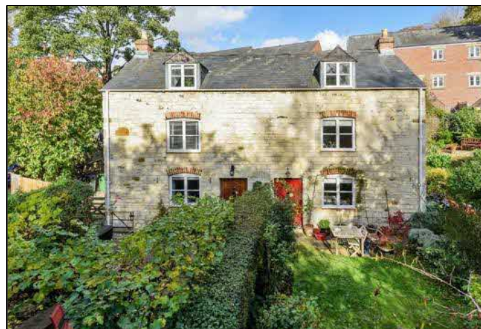
Plate 33: Cottages at Arundell Mill as viewed from the south. 19
