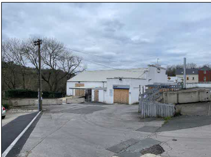
Plate 4: Southern parcel as viewed from London Road to the south-east.
